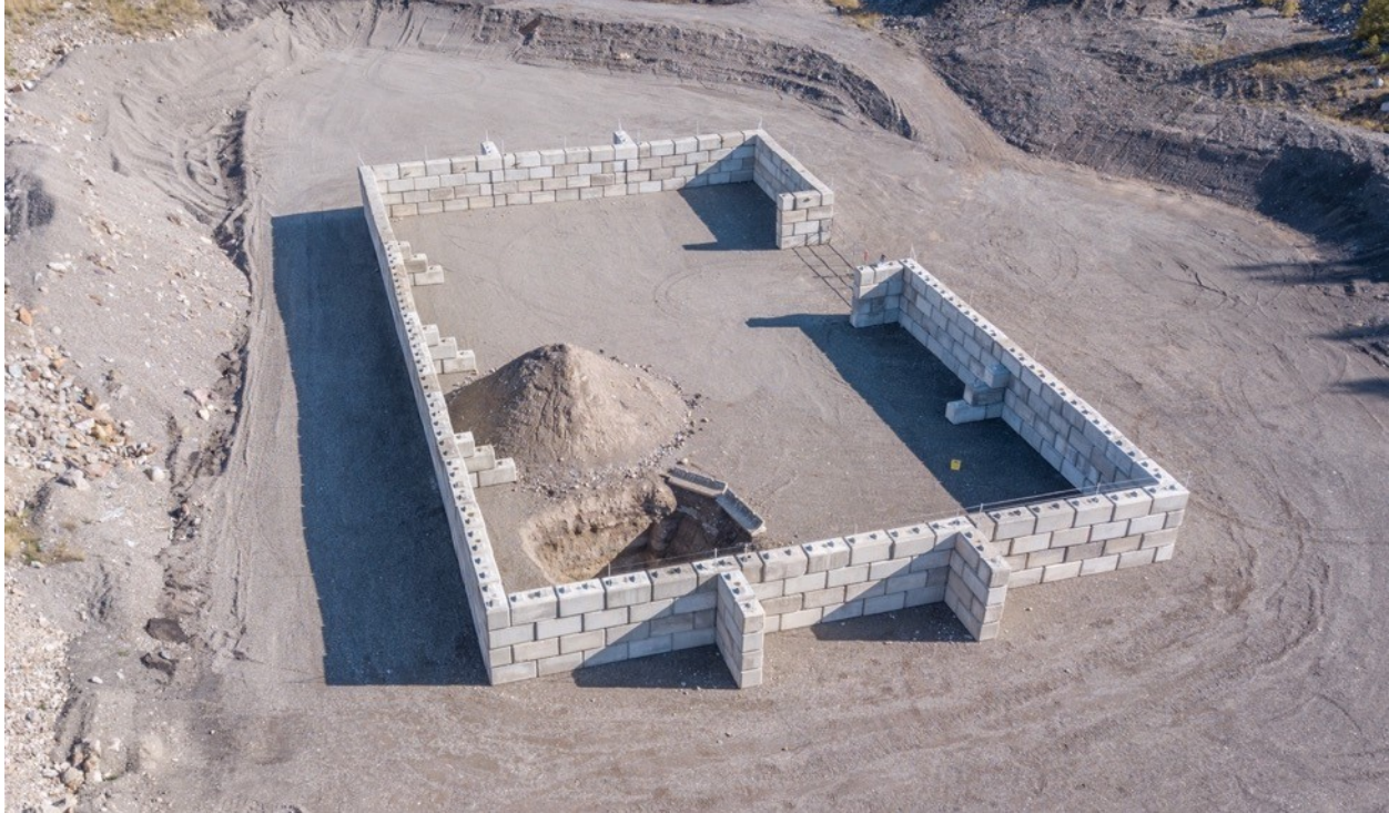
Figure 7-3. Enclosure built by BC's Ministry of Transport to aid in responsible disposal of roadkill carcasses. The enclosure is ~1600m 2 and is fully electric fenced and electric gated to ensure no entry of large carnivores.
