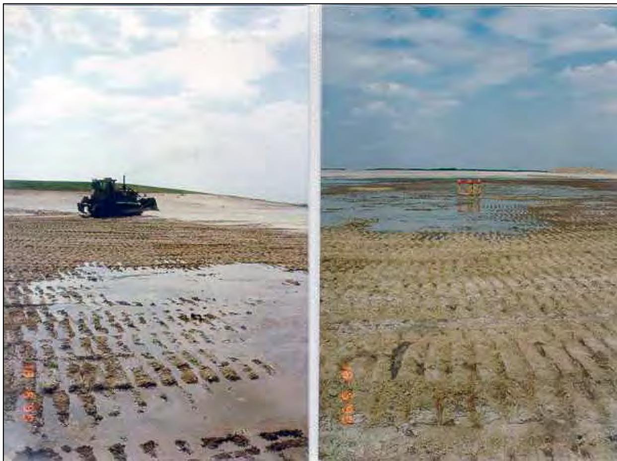
**Figure 4-8.** Mechanical compaction of 1-ha trial at the CT Prototype in 1999.
