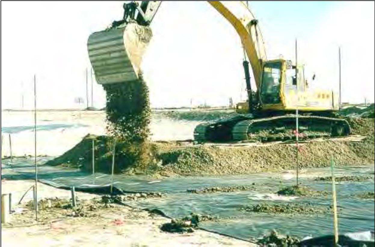
**Figure 4-2.** Loading of the trial embankment at the NST Field Demonstration U-Shaped Cell in 1999.
