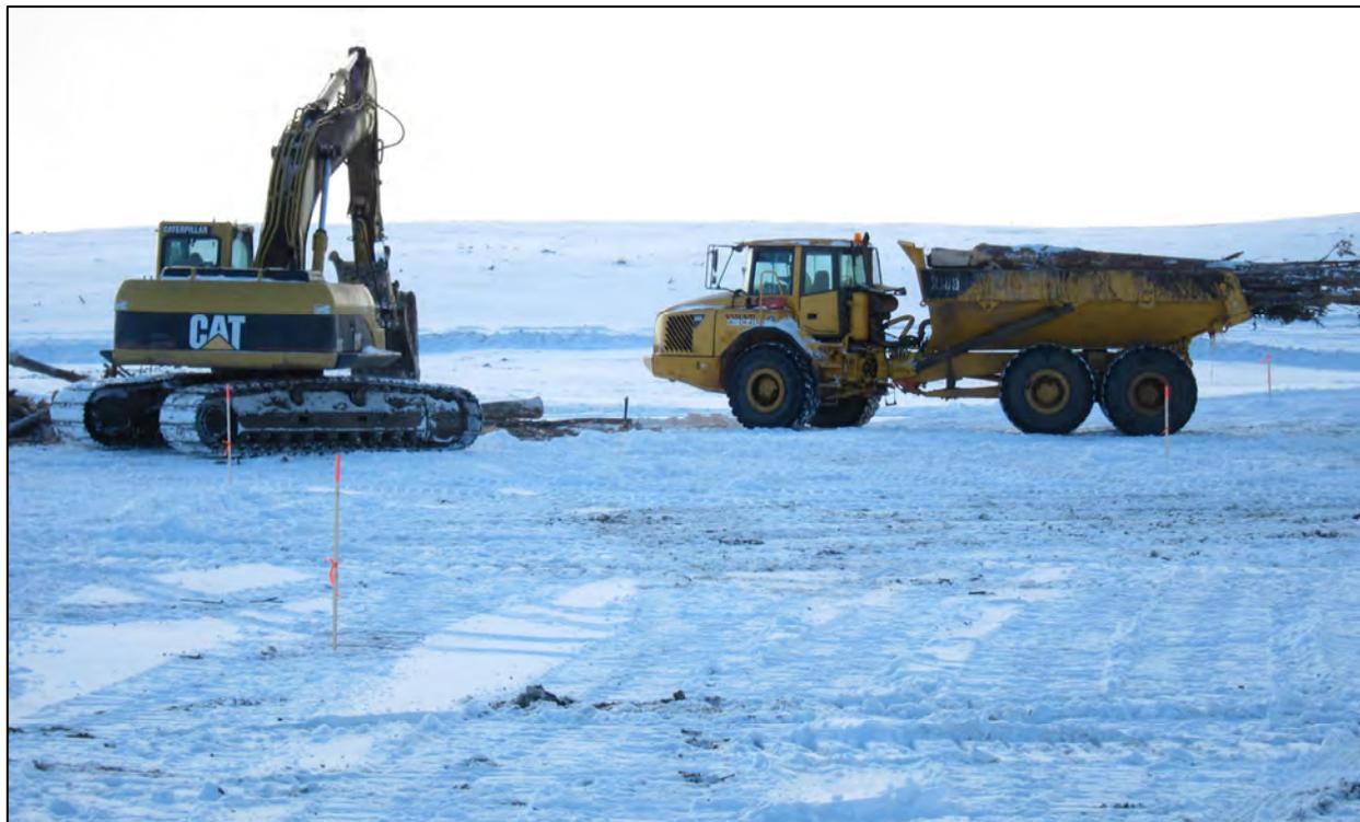
**Figure 4-16.** Winter placement of coarse woody debris at Sandhill Fen Watershed by mining equipment.
