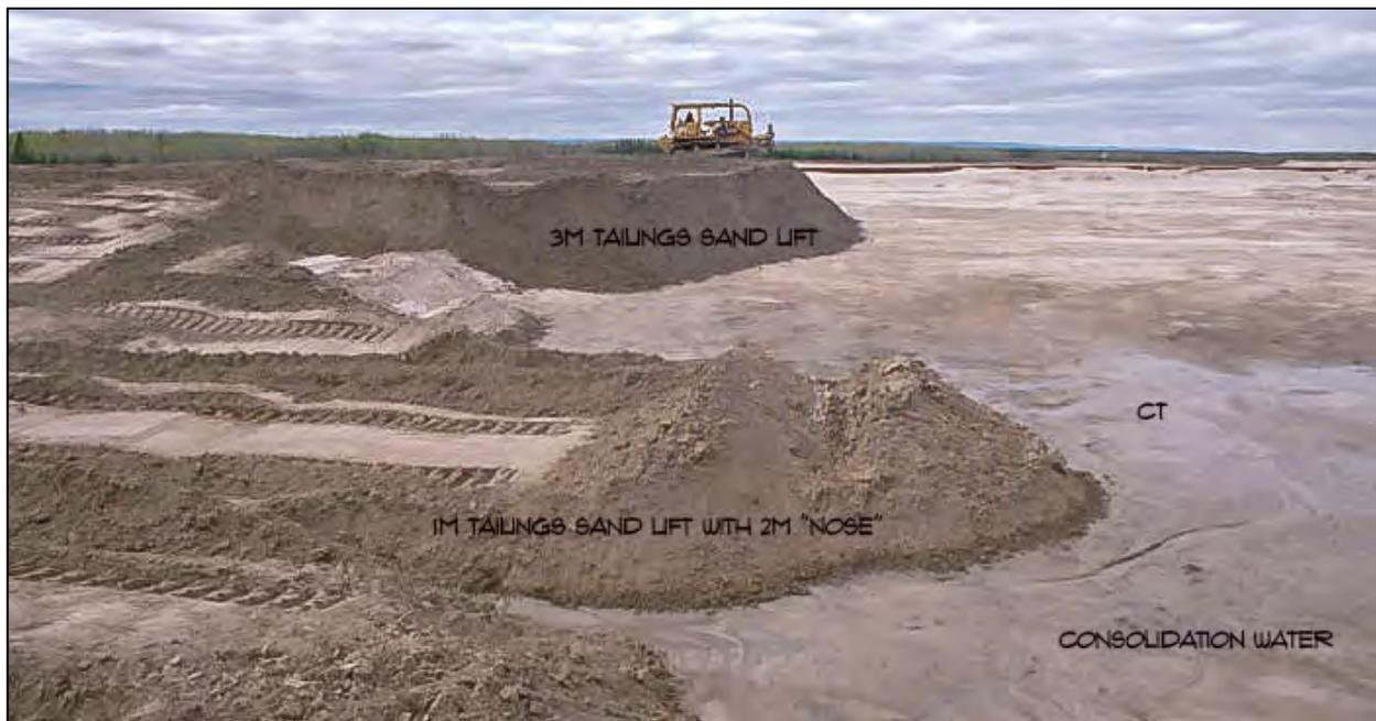
**Figure 3-5.** Mechanical placement of tailings sand on CT at Syncrude CT Prototype in 2000.
