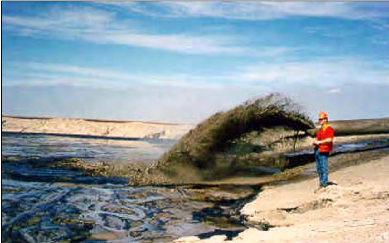
**Figure 4-7.** Hydraulic sand-capping of the CT Prototype in 1998.
