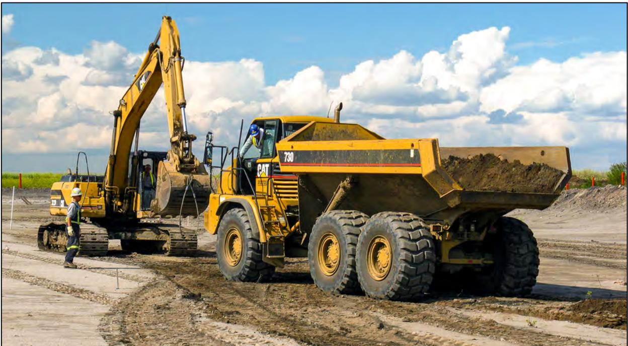
**Figure 4-6.** Trafficability testing on uncapped CT at the NST U-Shaped Cell in 2008.
