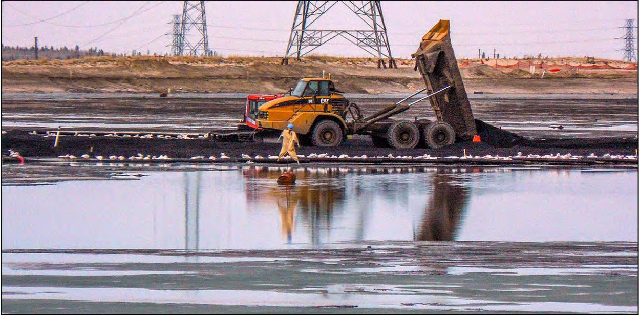
**Figure 4-19.** Placement of floating coke cap on Suncor Pond 5 off-spec CT.
