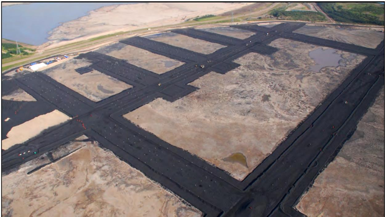
**Figure 1-7.** Suncor Pond 5 CT during initial floating coke cap construction.
