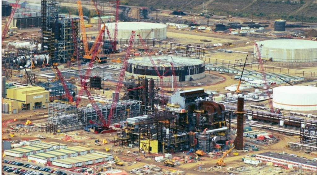
Figure 4.2: A typical modular site
