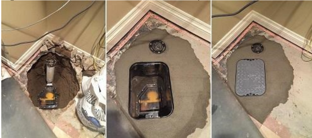
Figure 3: Backwater Valve Installation Example
