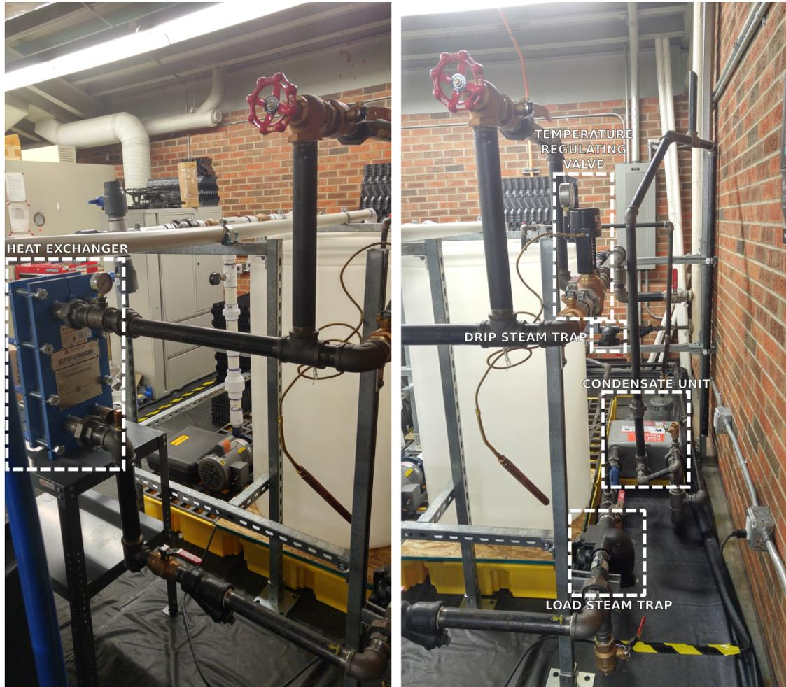
Figure 3.3 – Steam heating system as installed
