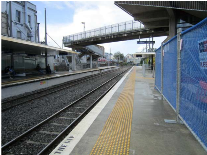
Figure 2.3: Construction at Kingsland Station showing pedestrian bridge over rails - May 2010.
