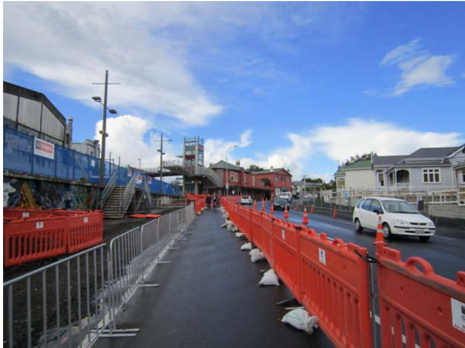
Figure 2.4: Construction at Kingsland Station - May 2010. Source: Author.
