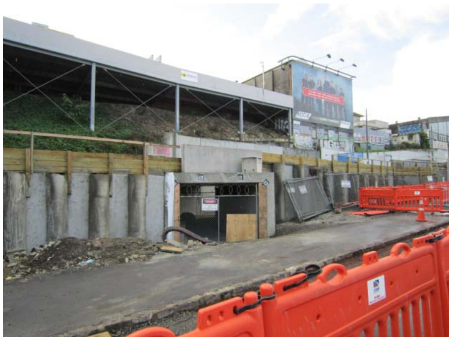
Figure 2.5: Construction at Kingsland Station showing pedestrian underpass - May 2010. Source: Author.
