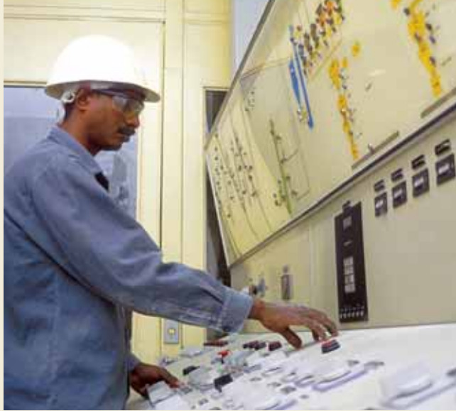
Norival Cezário, Mineral Salt Operator, works in the control room at our Brazilian feed plant.
