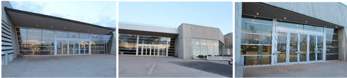
Figure 24: Photographing Entrances to the CWM.
