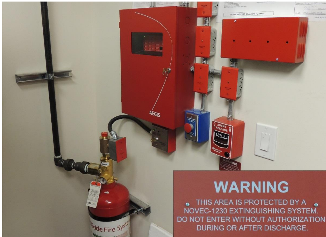
Figure 8: Chemical-based Fire Suppression System
