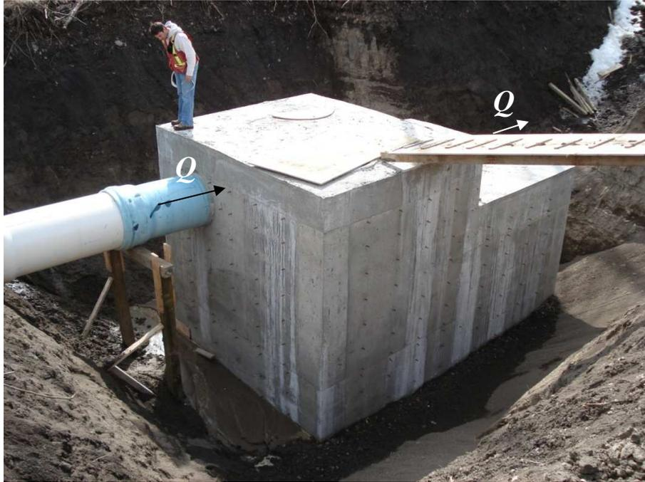
**Figure 2.1** Constructed stacked drop manhole in Windermere, Edmonton. A total of 5 such manholes were used to resolve an elevation drop of 50 m.
