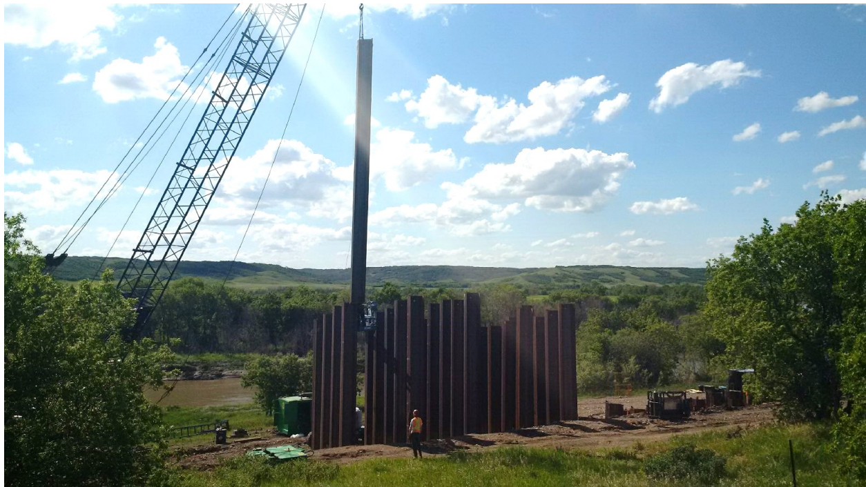
Figure 3.13: Hoisting sheet pile with crane (Source: CN).
