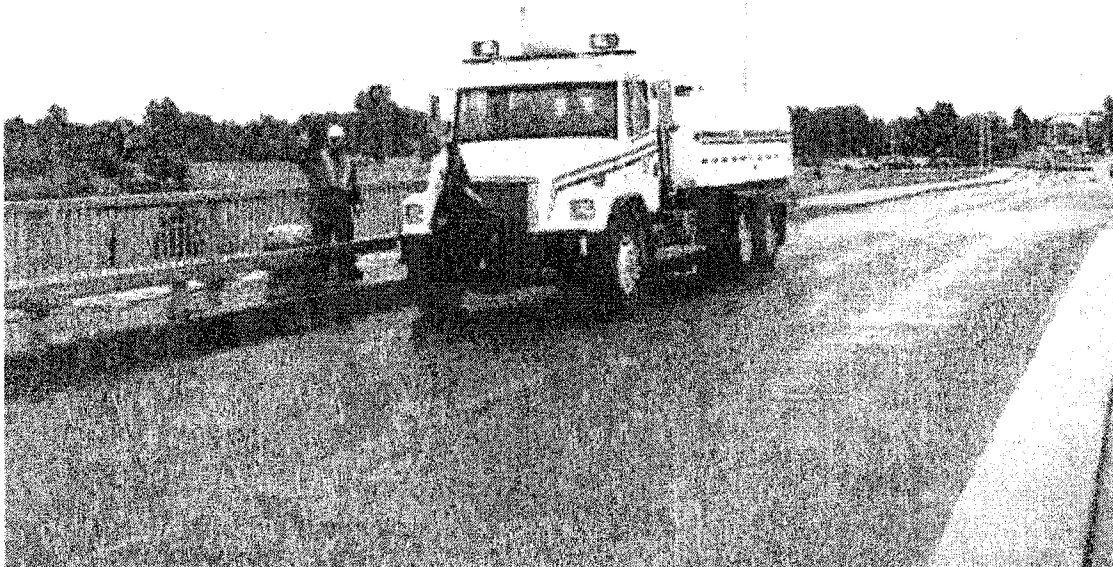
Figure 5.78: Static & Dynamic load tests with truck load
