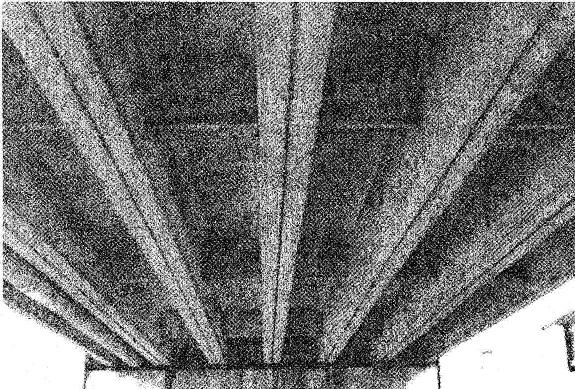
Figure 5.71: View of underside of the bridge
