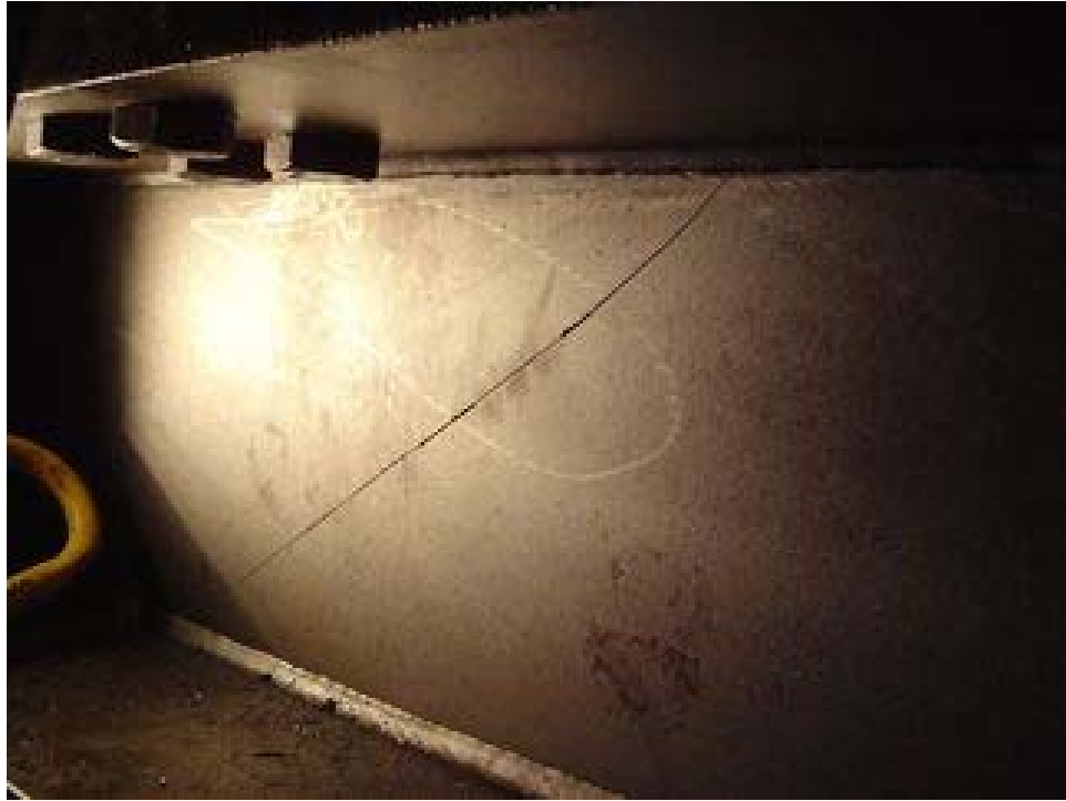
Figure C.1 – Diagonal crack in reaction beam under North actuator.
