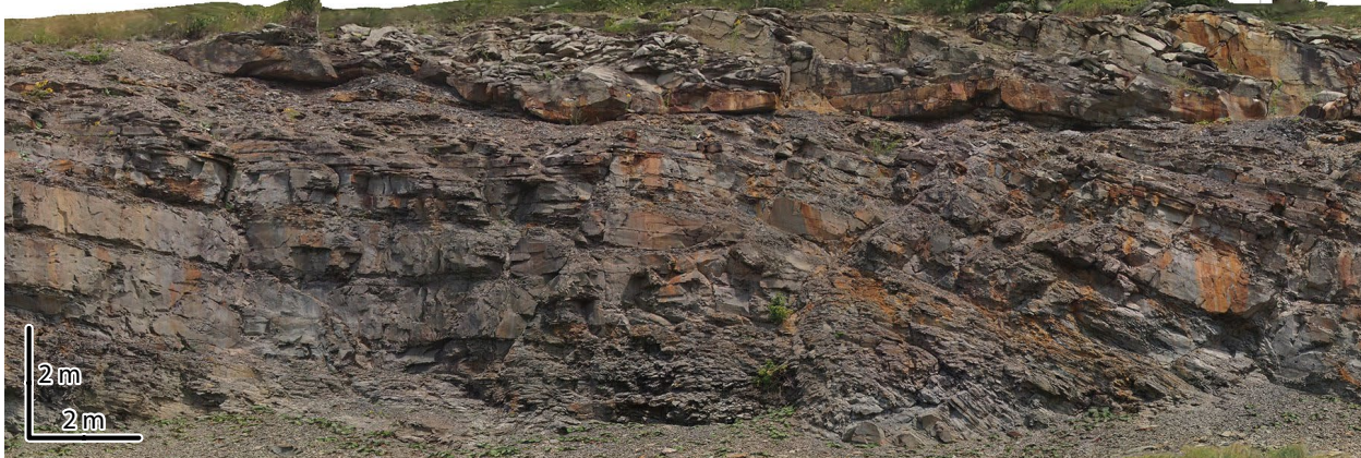
Figure 2.10. A small portion of a vertical orthomosaic photograph of the northern roadcut.
