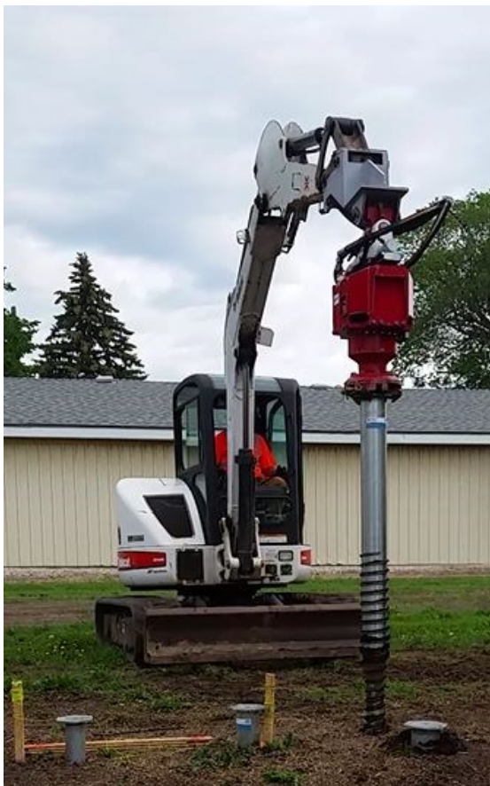
Figure 4-7: Photo of a steel threaded micropile during installation.
