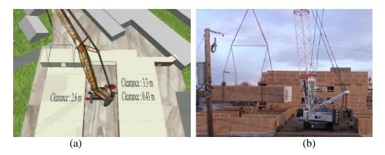
Figure 4.11: Crane clearances: (a) visualization model, (b) construction site
