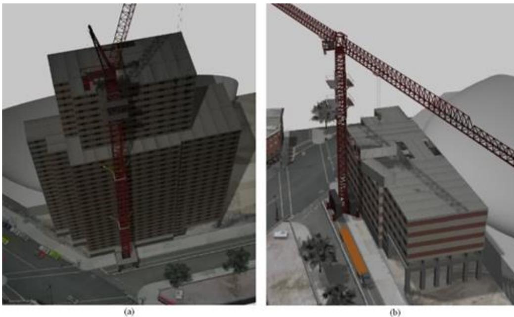
Figure 4.13: 34-storey modular building construction using (a) single-jib tower crane, or (b) double-jib tower crane
