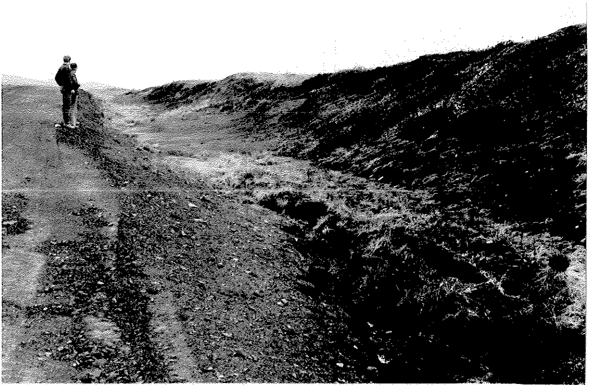
PLATE 19: Slumping of cut in ice-rich silt.
