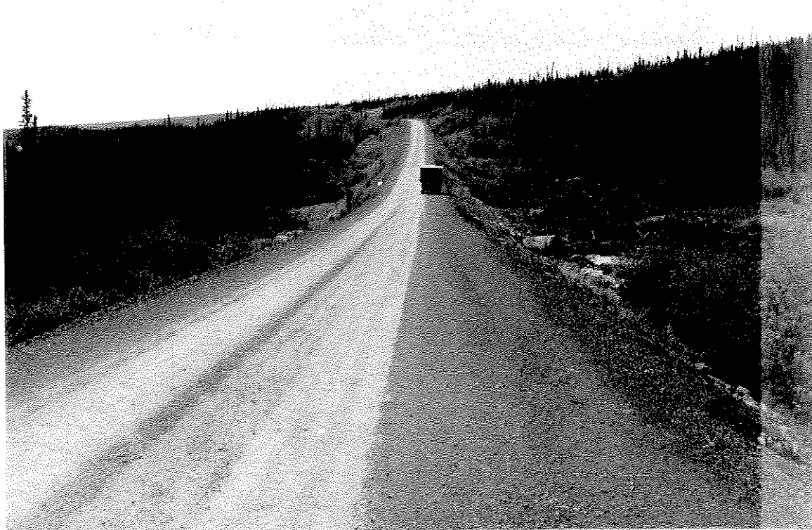
PLATE 2 : Spruce forest/sphagnum moss plant association. "Broken back" culvert in a deep fill (centre). Remnant aufeis and icing area visible (right). (Kilometer 29)
