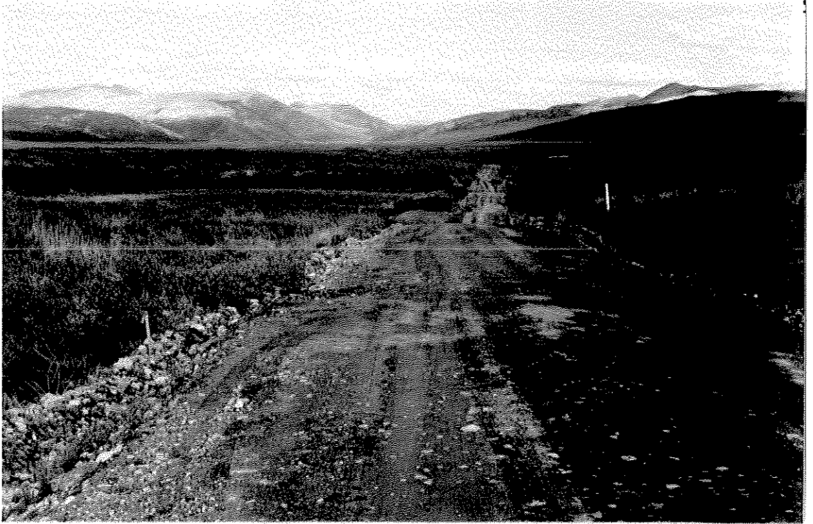
PLATE 7: Looking north from Km. 122 (Built 1962). Surficial soils consist of 0.1 - 0.5 m. of saturated organics overlying ice rich silts or sands.
