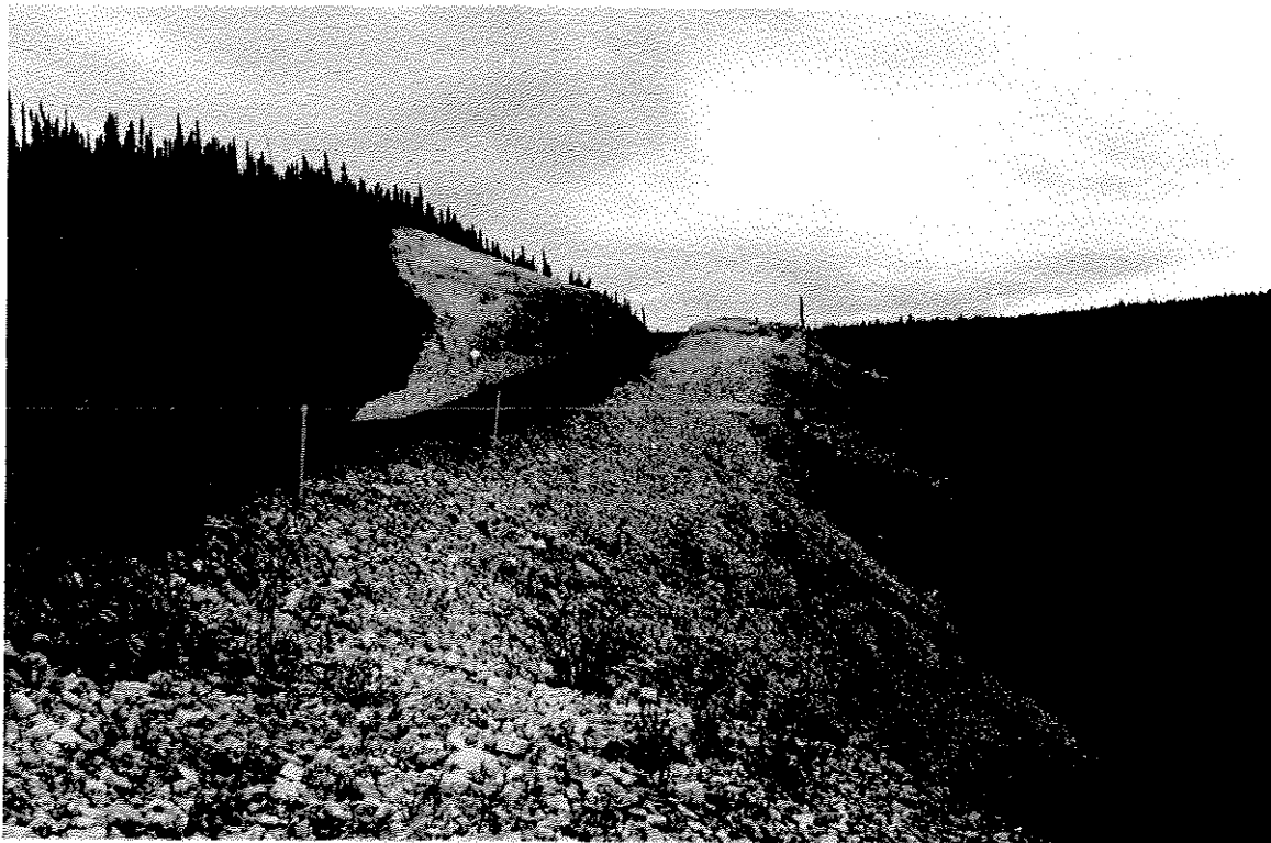
PLATE 11: Cut/fill transition at Km. 354. Limestone breccia in rock cut.
