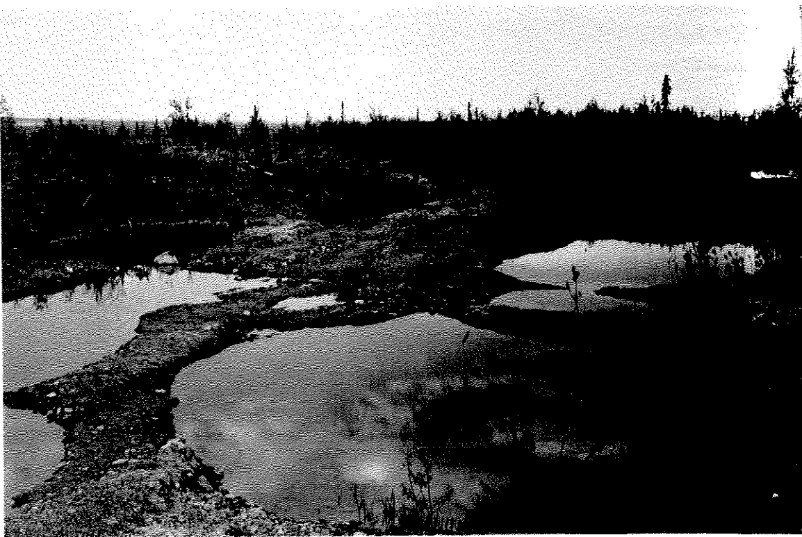
PLATE 26: Borrow pit at Km. 720. The sinkholes (about 5m. across) resulted from thaw of ground ice. A polygonal pattern has developed.
