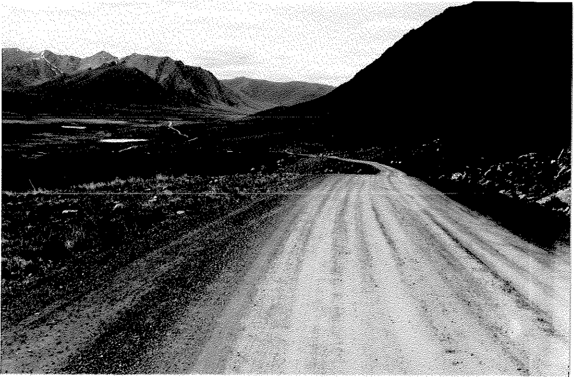
PLATE 5: Highway reconstruction underway near Km. 81 in alpine "tundra" of the Ogilvie Mountains (looking north). Remnant aufeis is visible at the left.
