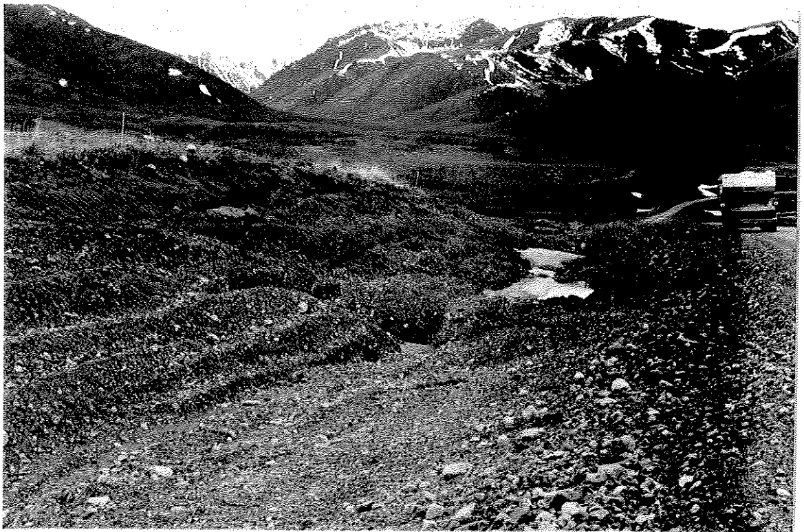
PLATE 6: Backslope cut at 28 degrees to the horizontal in silty sand. See Figure 14 for cross-section. (Km. 87)
