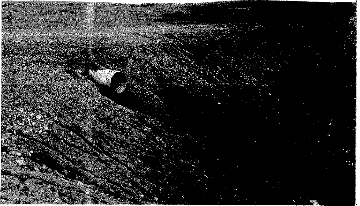
PLATE 21: No flume on culvert. Consequent erosion is considerable. (Km. 510).
