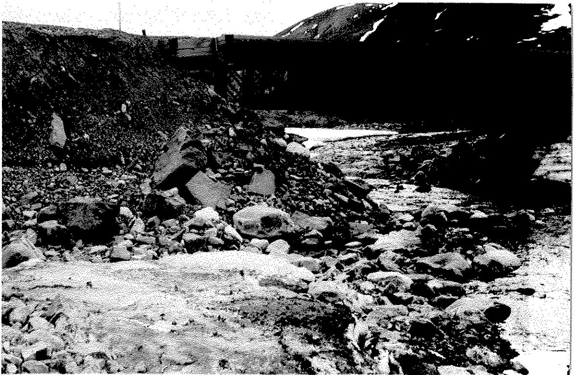
PLATE 4: Overdeck Bailey bridge at Blackstone River. Remnant aufeis (right) is almost at truss level. (Km. 78)
