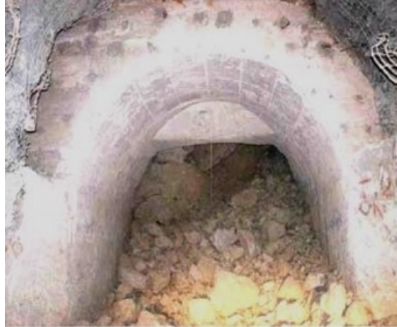
Figure 2.6: Fragmentation of caved material at a drawpoint, Rubio (2006)
