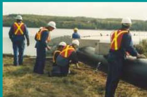
Pipeline then weighted and fed out from shore and joined to vault with control valves.
