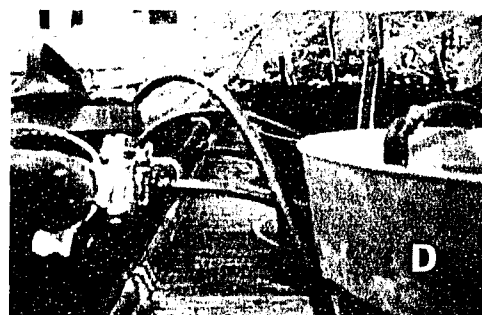
Figure 2-1. Greenhouse before bioassay plant production (A) and detail of automated watering system: watering timer and solenoid valve control (B), solenoid valve intersecting water supply (C), and drip irrigation spikes, fed by main water line and inserted into soil (D).
