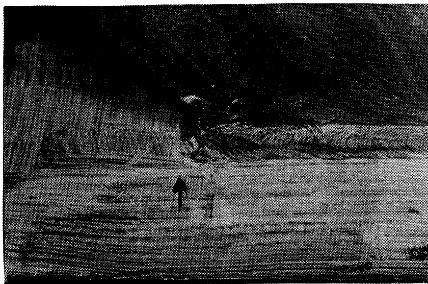
Figure 3.10 Fatigue Crack in Joint L1 (T2F)
