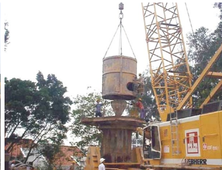
b) Load Concrete to Pile
