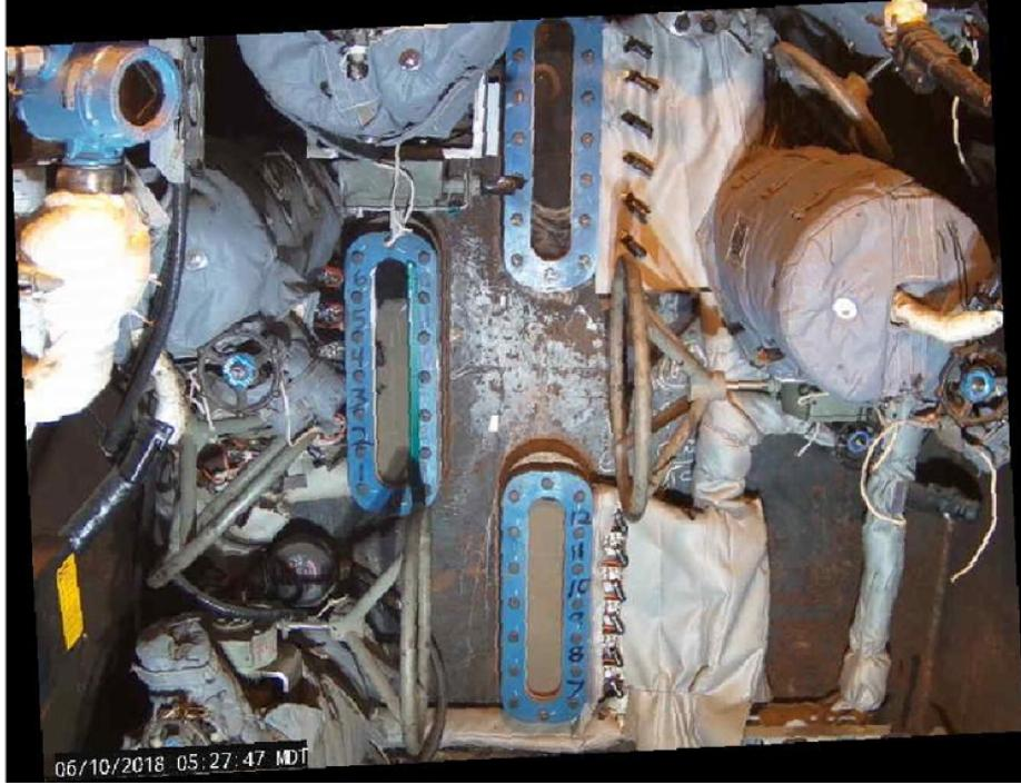
**Figure 4.6:** *Acquired image from video device mounted on PSV sight glasses.*
