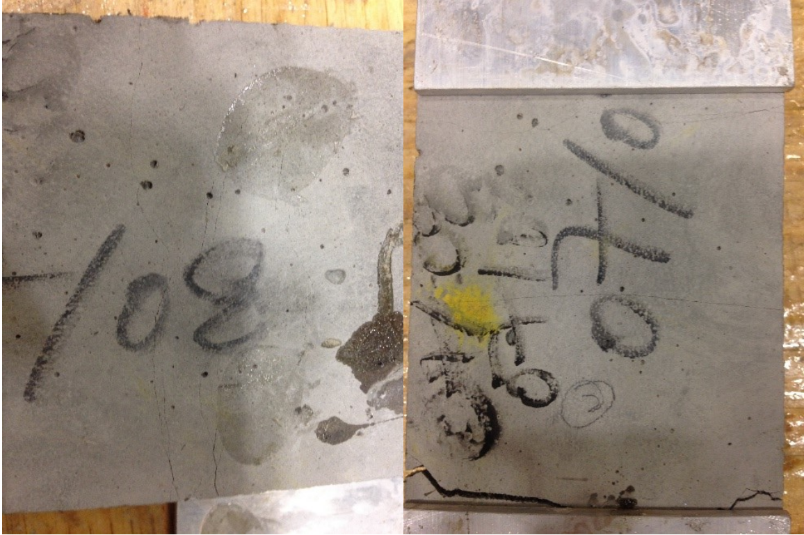
Figure 3-13: Tensile cracking on ECC02 coupon specimen
