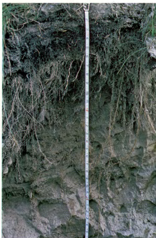
Plate 6. Penetration by roots of the grass cover on the dike shows that a very great percentage of the roots are concentrated within the peat layer at the surface. While this helps prevent erosion at the surface, washout of the dike is possible with heavy precipitation.
