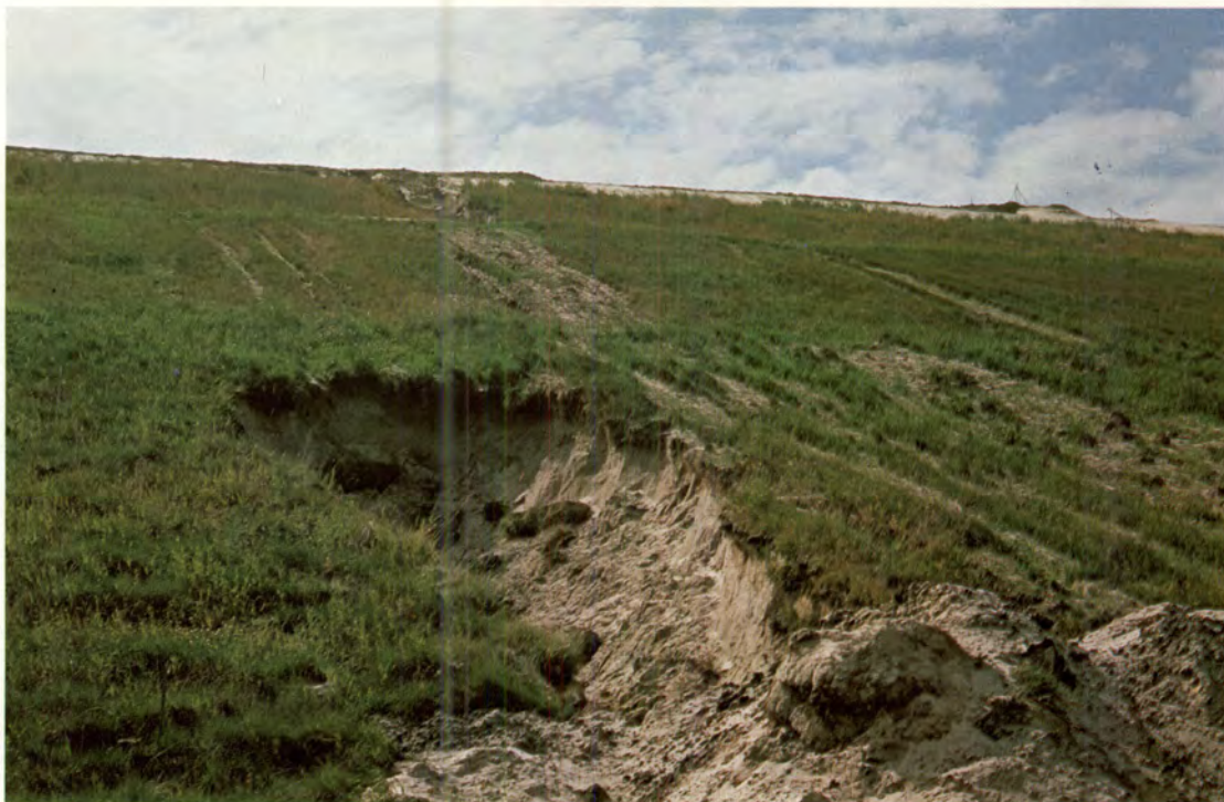
Plate 3. Once surface layer of organic matter is broken, erosion is difficult to control. Plate shows washout developing upslope from toe of G.C.O.S. dyke. Channel erosion and new dike construction are visible in upper portion of picture. Stabilization of upper slopes is crucial to protect vegetation on lower slopes.
