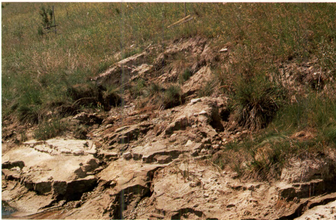
Plate 4. Tailings sand has a high infiltration capacity and permeability. Berms on G.C.O.S. dike influence surface and underground water movements, reducing channel erosion but contributing to seepage washouts such as this one.
