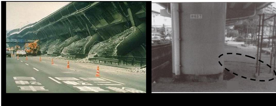
Figure 2.1. (a) Elevated road collapsed due to plastic hinging in the superstructure and (b) undamaged Pier 697 on Route 3 as the shallow foundation rocked during the same earthquake (Yashinsky and Karshenas 2003).
