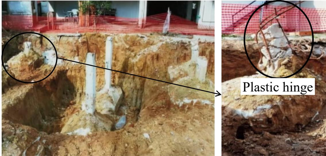
Figure 2.2. Columns and foundations of the one-storey building collapsed during moderate earthquake, 1999 Athens earthquake (Gazetas 2019).
