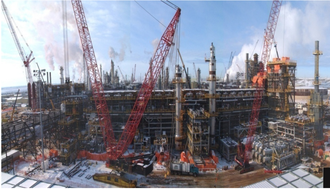
Figure 5-1 A typical congested industrial plant
