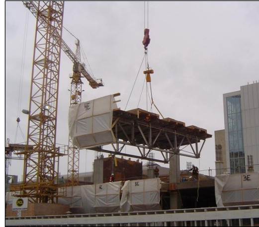
Figure 3. High-flyer formwork
