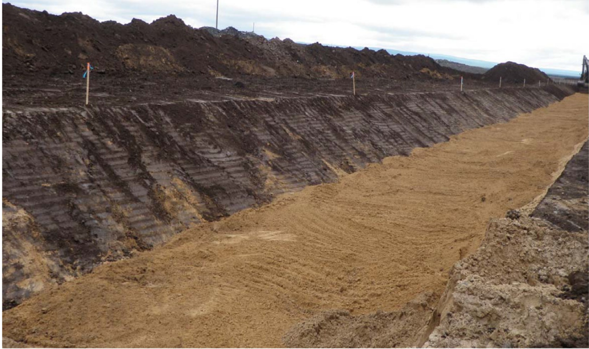
Figure 20. Chimney Drain Construction
