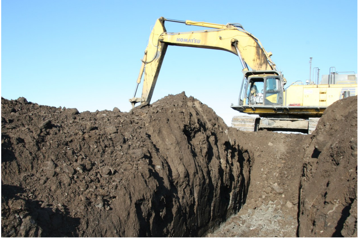
Figure 17. Trench excavated for a test fill. (CNRL, 2018)
