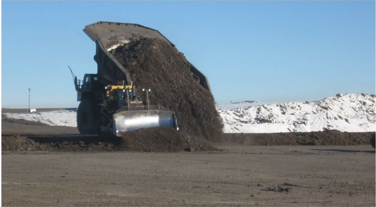
Figure 18. Fill placement while dozer spreads fill (CNRL, 2015)
