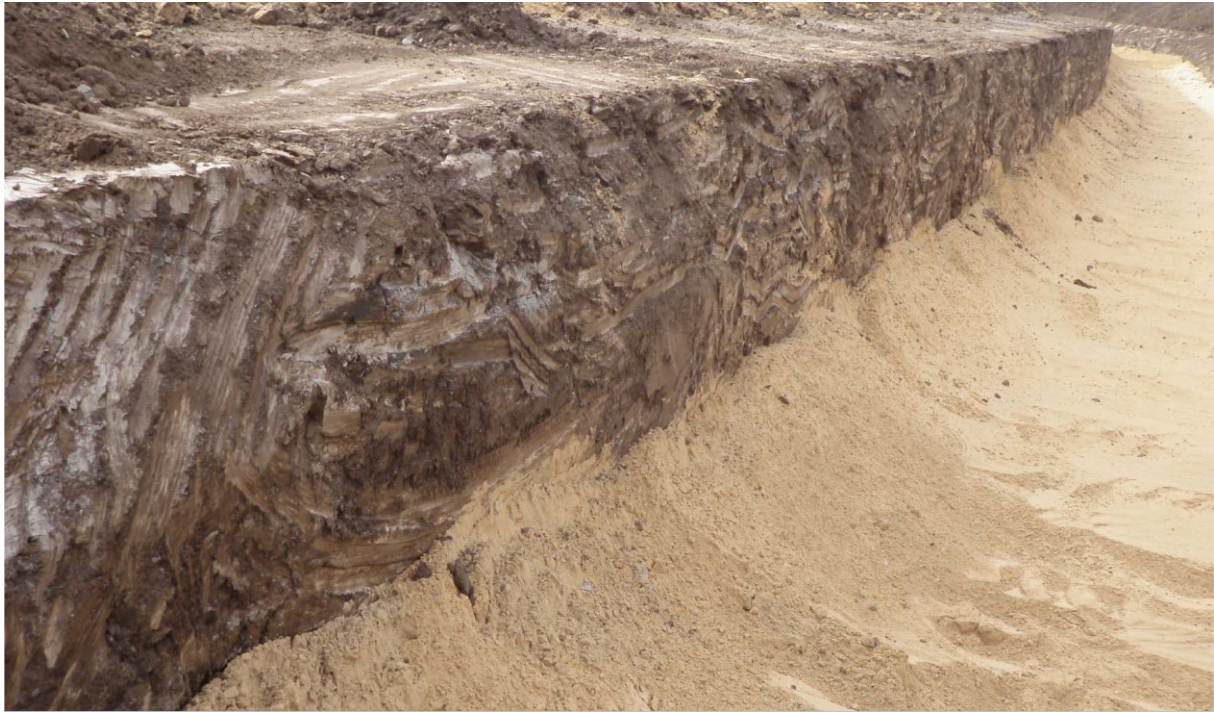
Figure 21. Chimney Drain Trench Excavation Exposing Compacted Lift (CNRL, 2018)
