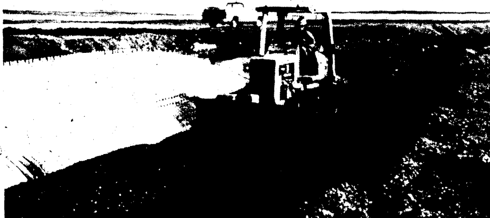
Figure 4.3 Compaction Beside the Prototype Arch-Beam Culvert
