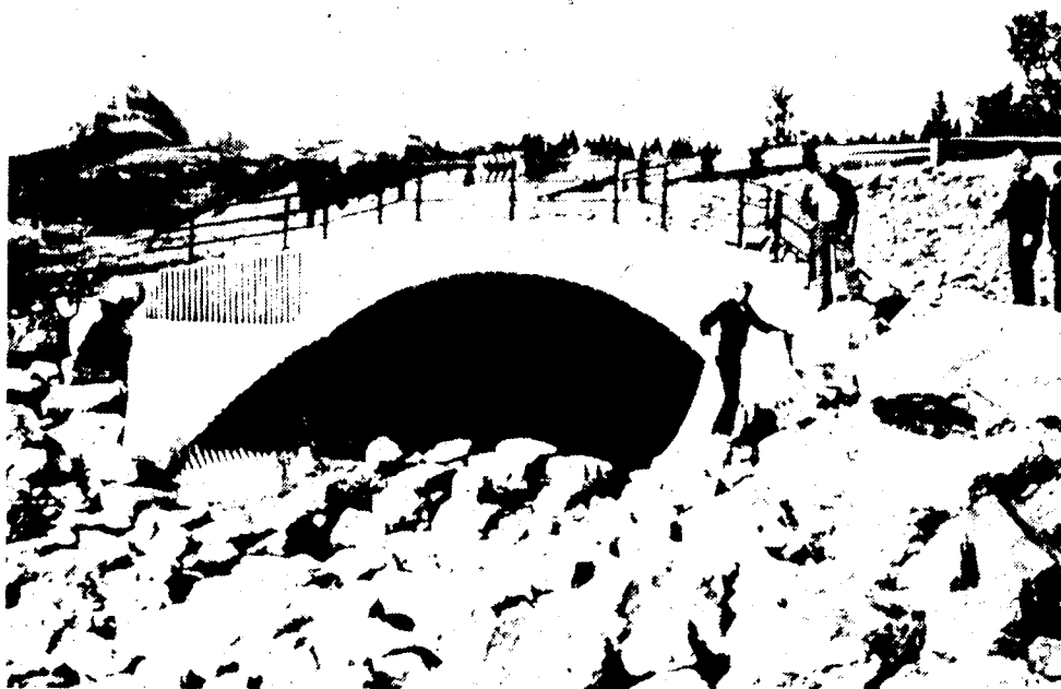
Figure 4.2 Blairmore Creek Arch-Beam Culvert
