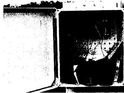
Tower details - datalogger box
