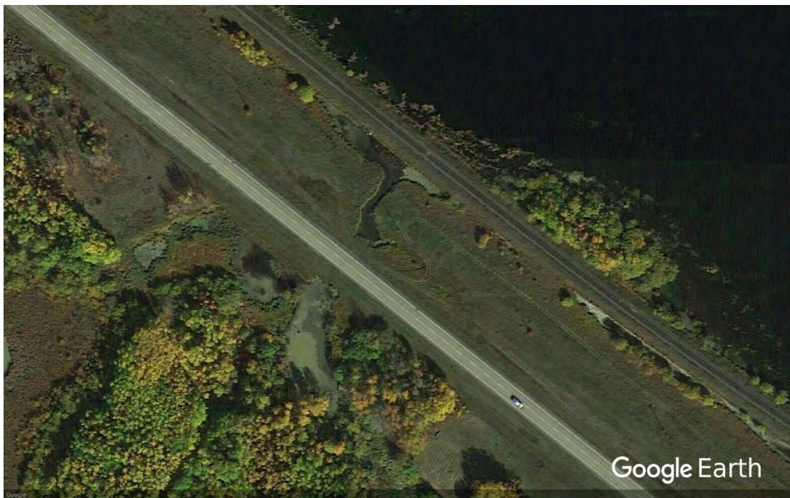
Figure 2.2 - Photo Showing Crossing From Little Antler Lake Under CPR Tracks and Standing Water before and after Wye Road Crossing.
