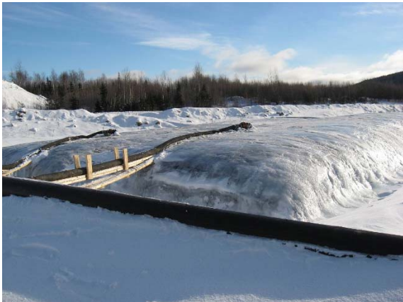
Picture 3: Geotube® containers in operation during winter.
