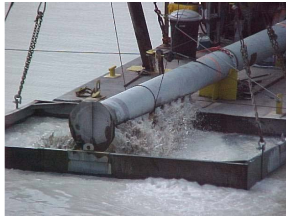
Figure 5. Surface diffusion of hydraulically delivered sand, raining sand through the water column to gently place it on soft tailings.
