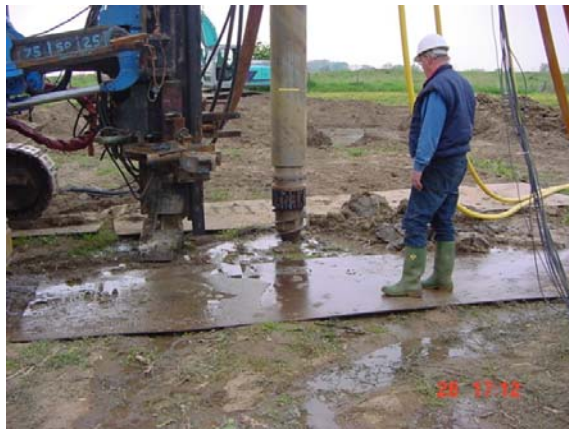
Figure 3. Subsurface dredging pilot test
