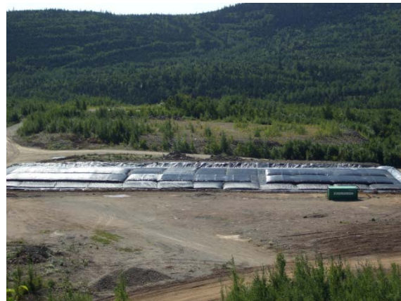
Picture 1: Pad with geotextile containers.
