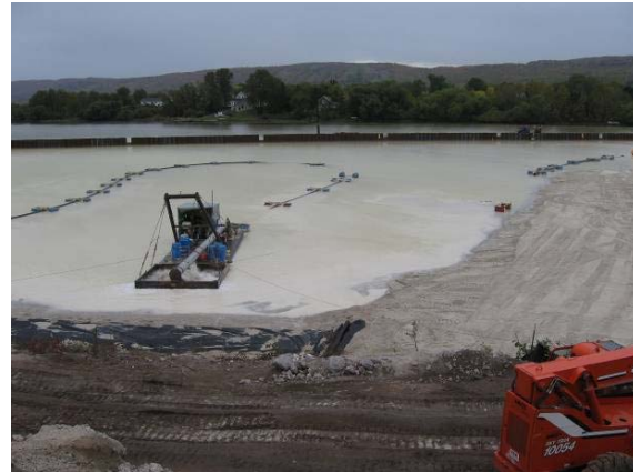
Figure 11. Surcharge cap installation at Stryker Bay.
