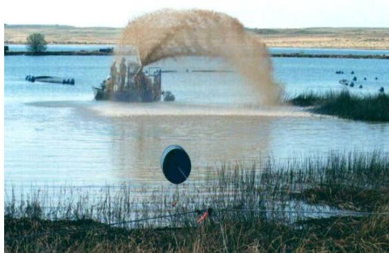
Figure 7. Rainbowing sand from a slurry cannon. (Thompson 2003)
