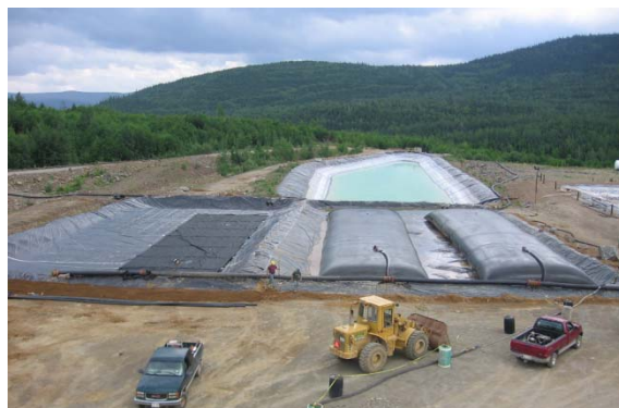
Picture 2: Geotextile container set up for filtration in a flow process.
