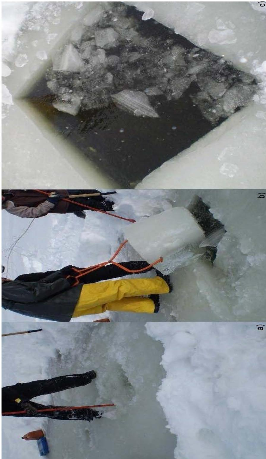
FIGURE 2-6 a) The ice blocks are loosened using an ice pick; b) The ice blocks are removed using ice tongs; c) The 1m X 2m section is free of ice once all the ice blocks are removed
