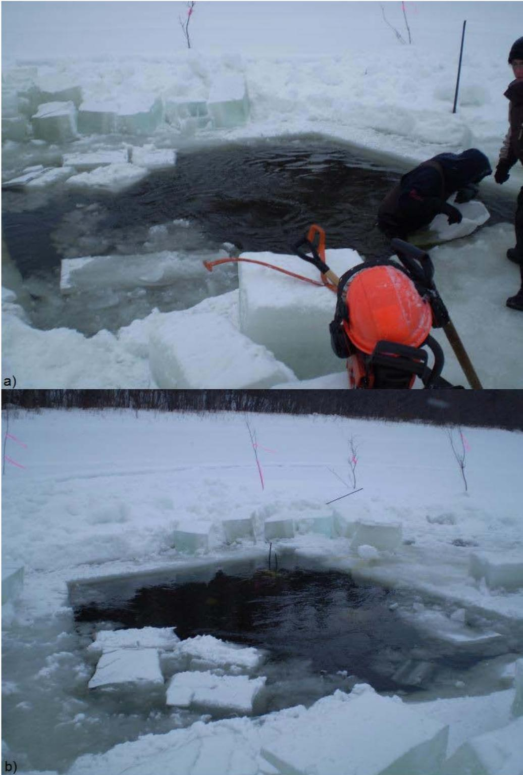
FIGURE 2-7 a) and b) Two photos of a 3m X 4m section free of ice in the Athabasca River following sawing the section into ice blocks using a chainsaw and removing the ice blocks using ice tongs and placing them around the section
