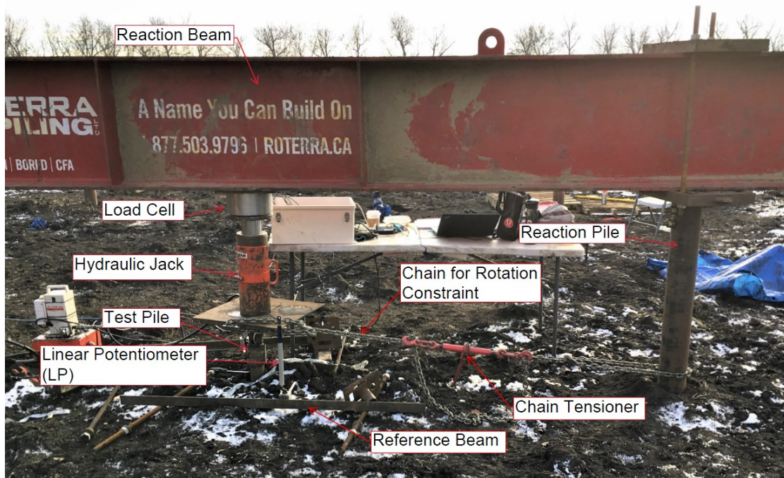
Figure 3-7. Load test setup photo.
