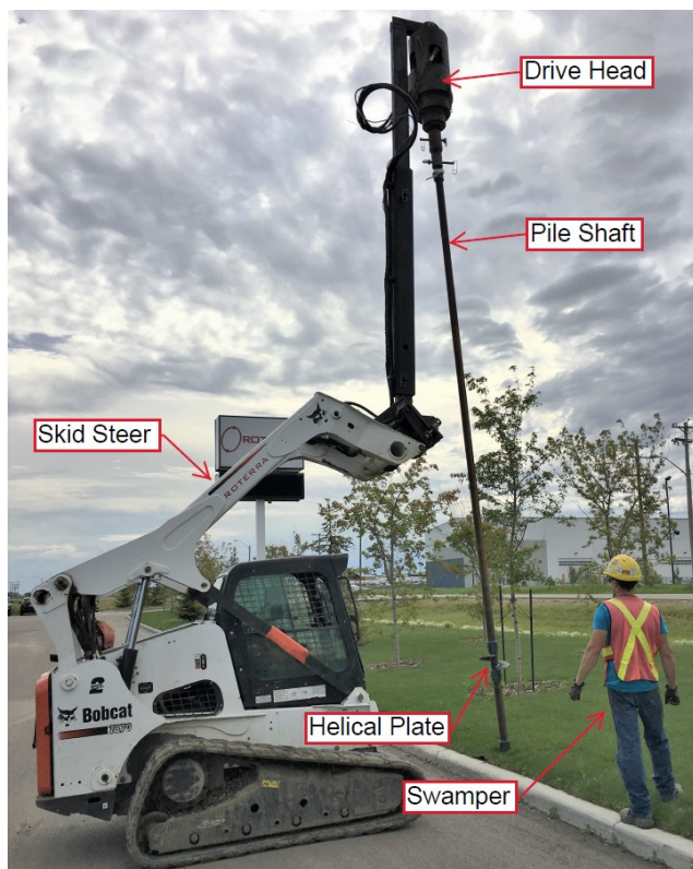
Figure 1-2. Typical helical pile installation.
