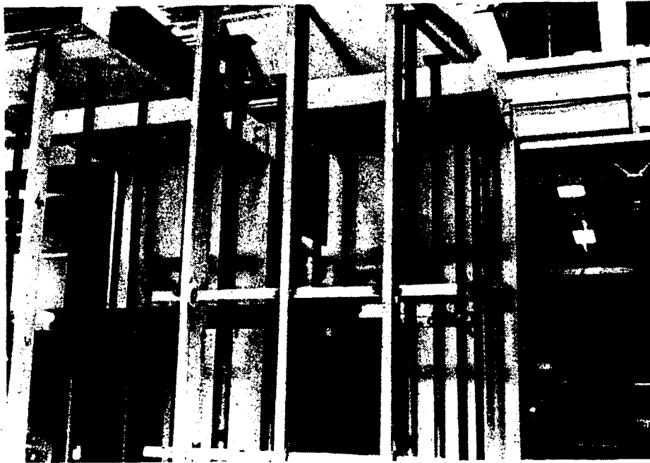
Figure 3.11 Full Sized Wall Studs and Bridging Assembled
