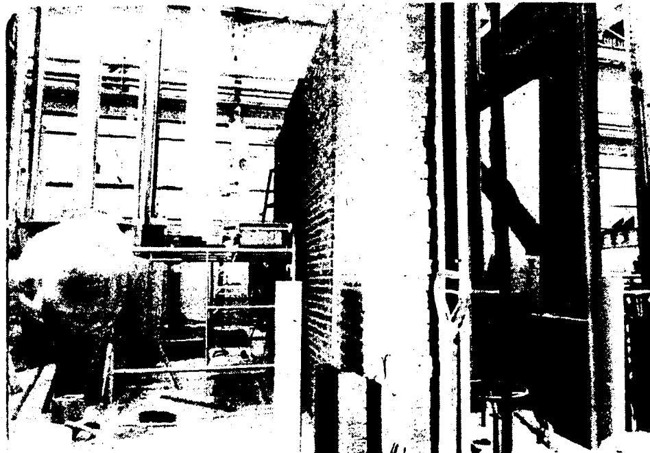
Figure 3.14 Full Sized Wall Specimen Completed
