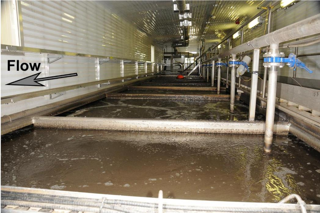
Figure 2-2: Representative image of a functioning aeration tank in the WWTP examined in this study. The camera is located at the upstream end of the tank (opposite end from the anoxic zone). The arrow points in the direction of the flow of process fluid.
