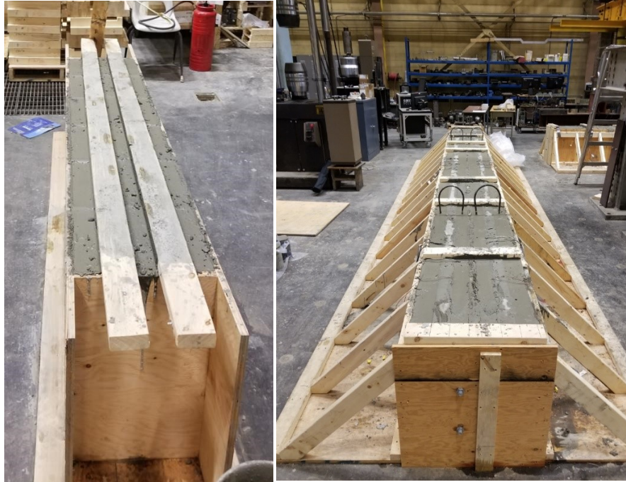
Figure A.8 Specimens immediately before curing (a) push through formwork (b) full panel formwork
