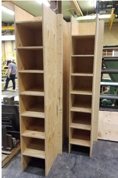
Figure A.1 Push-through formwork
