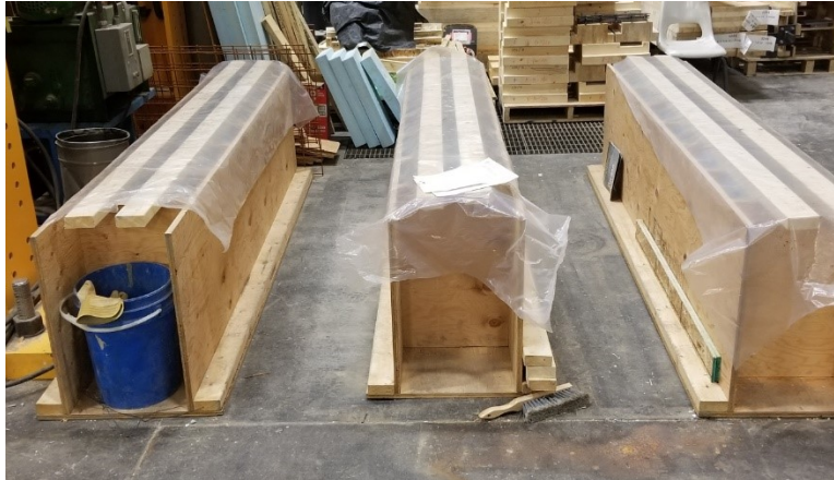
Figure A.3 Formwork preparation
