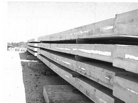
Figure 2.14 Concrete wall panels in storage (Losch, 2003)
