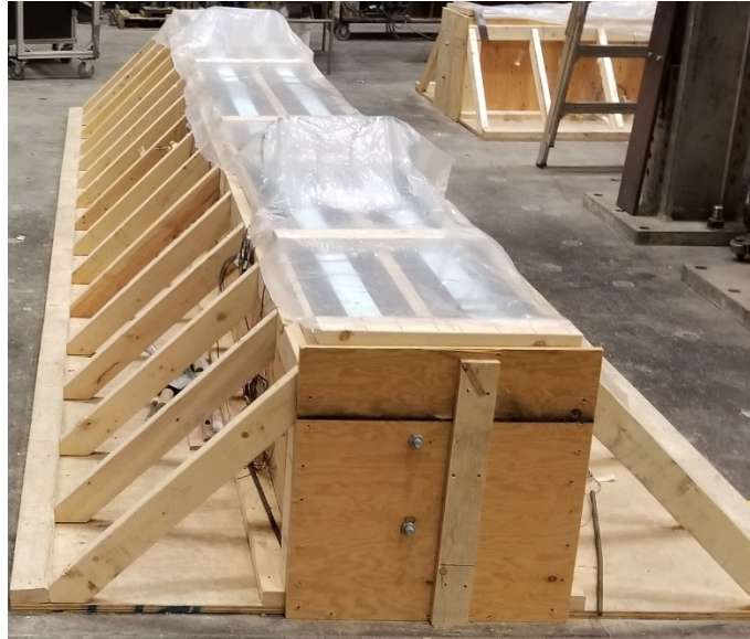
Figure A.5 Formwork preparation
