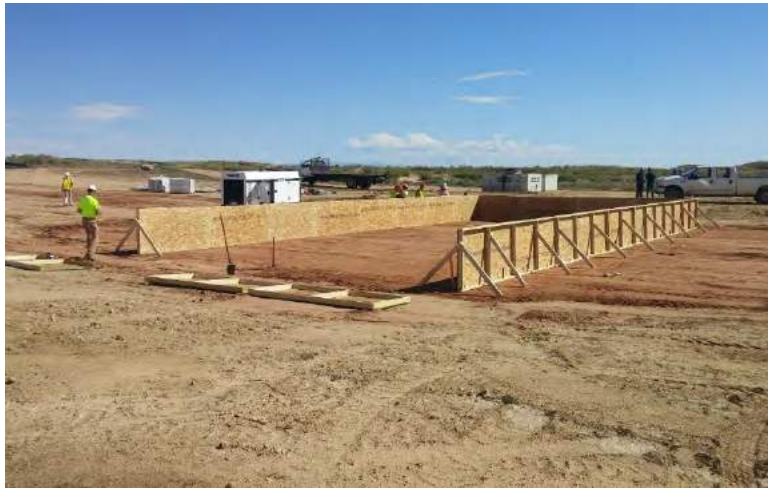
Figure 4. Lysimeter formwork installed for first stage and prior to deploying the geomembrane.
