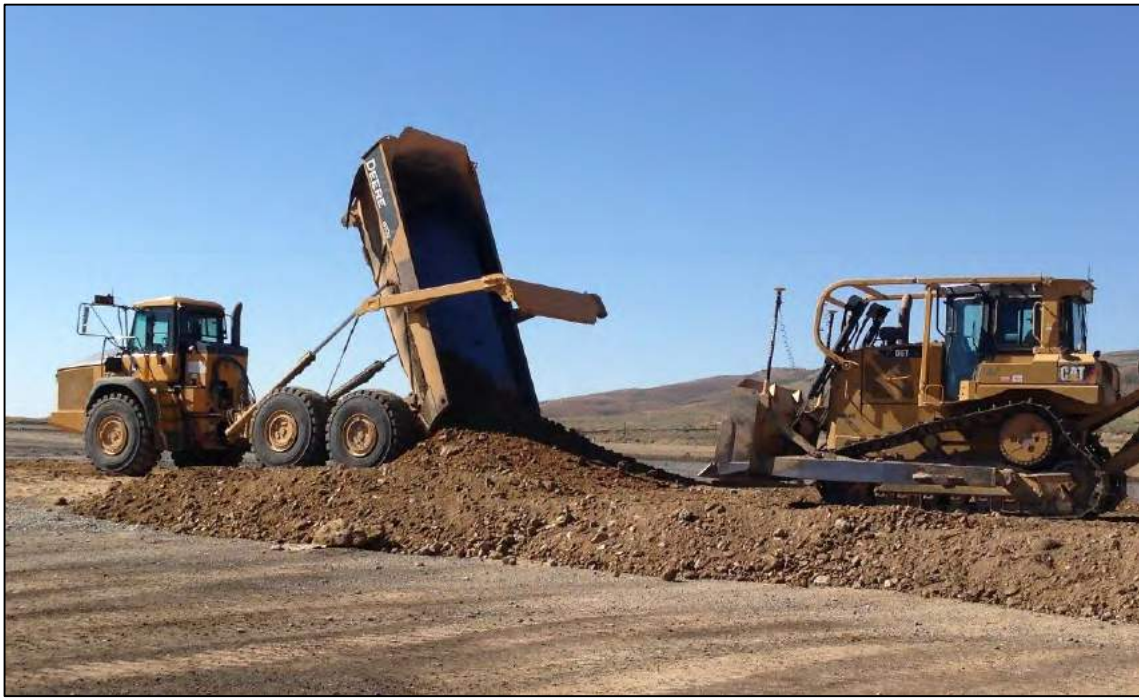
Figure 17. TSF 1 interior contour berm construction.
