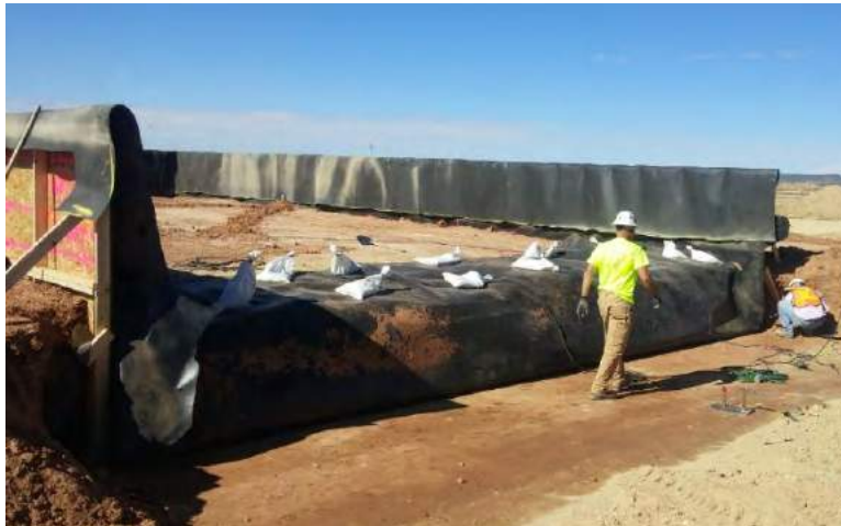
Figure 6. Folding up and welding geomembrane on the upslope end of the lysimeter after placement of the cover soils during the first stage. A technician is extrusion welding the northwest corner (right side of photograph).
