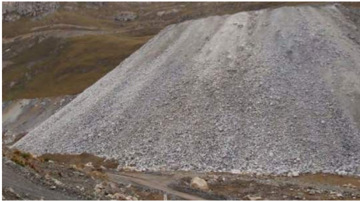
Figure 4. Rock drain created by end dumping method (Hawley & Cuning 2017) photo by J. Hogarth.
