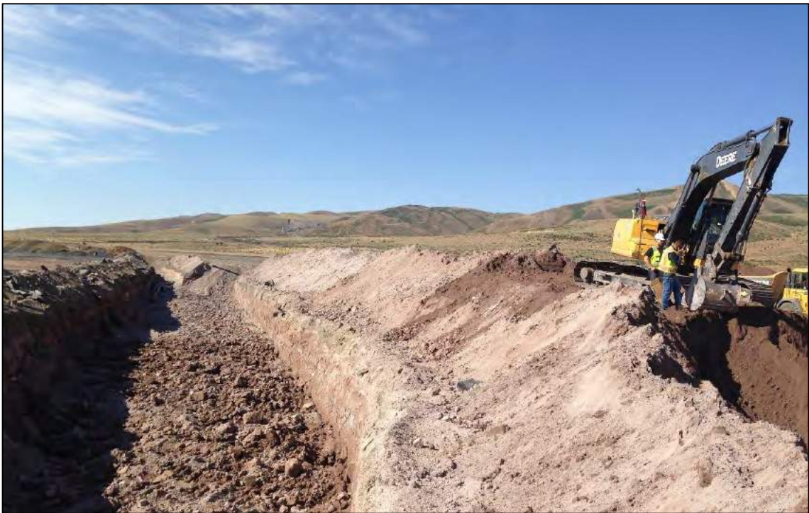
Figure 13. Excavating and hauling dried tailings.
