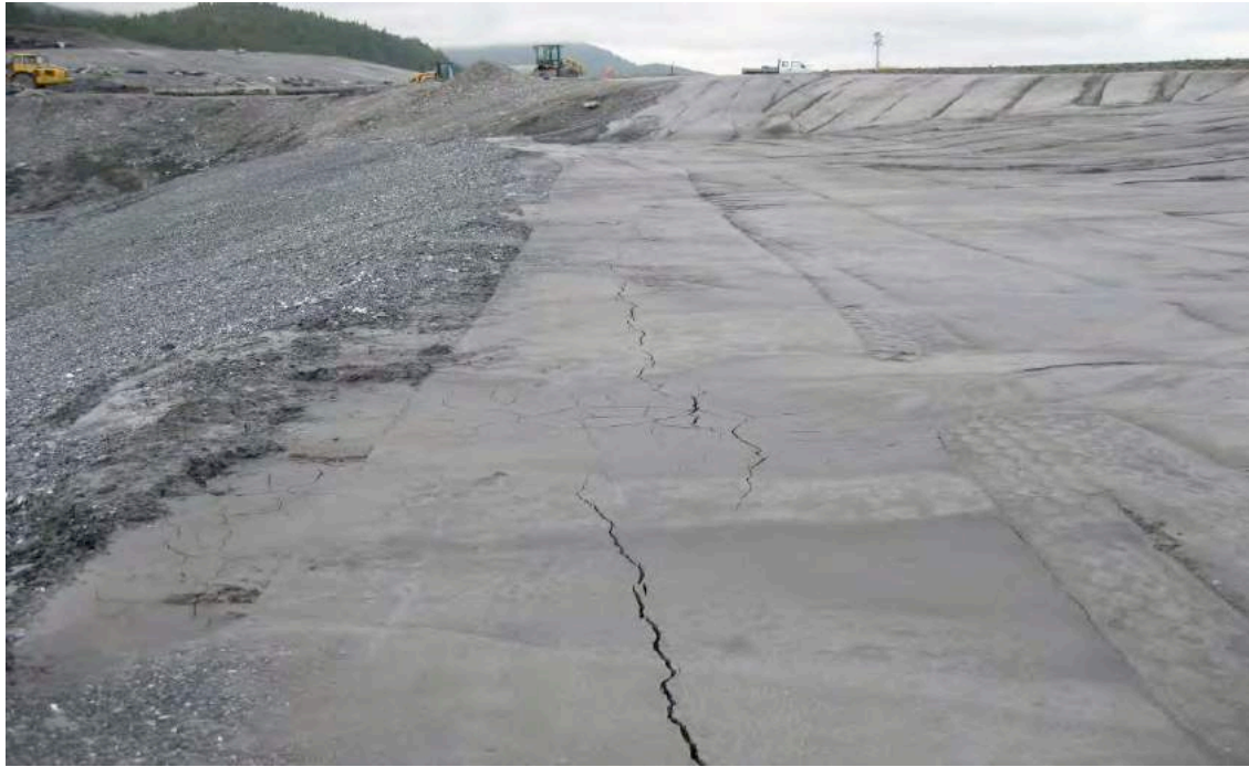
Figure 6 Cracking because of placement of wet material
