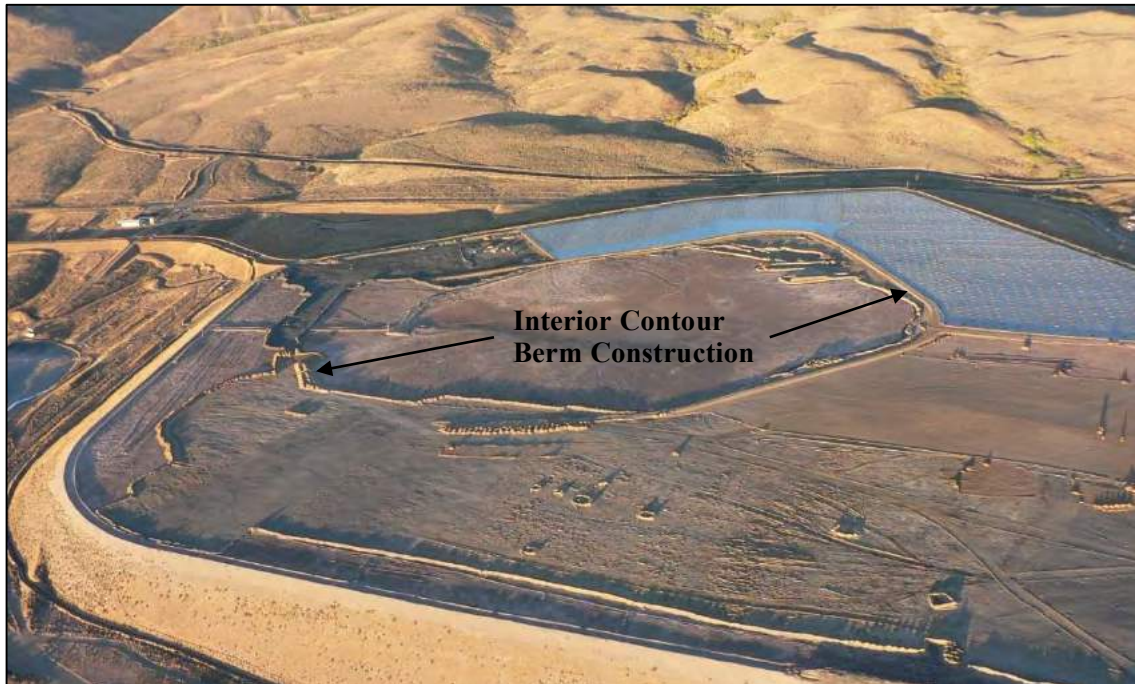
Figure 16. TSF 1 interior contour berm construction (looking west).
