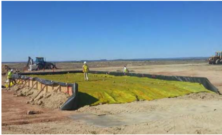
Figure 7. Deploying root barrier (yellow layer) over the interim layer.
