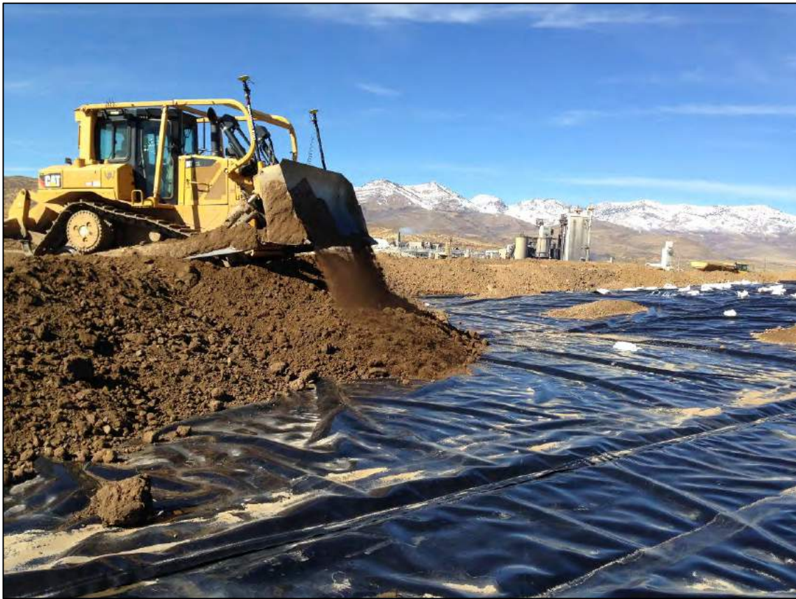
Figure 22. Growth media placement over geomembrane liner
