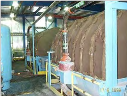
Figure 3. Vacuum disc filter. Source: Confidential client.
