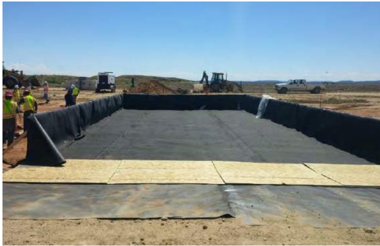
Figure 5. Geosynthetic drainage layer after placement during first stage of construction. Plywood panels were placed to protect the geomembrane upslope of the lysimeter during placement of the cover soils.
