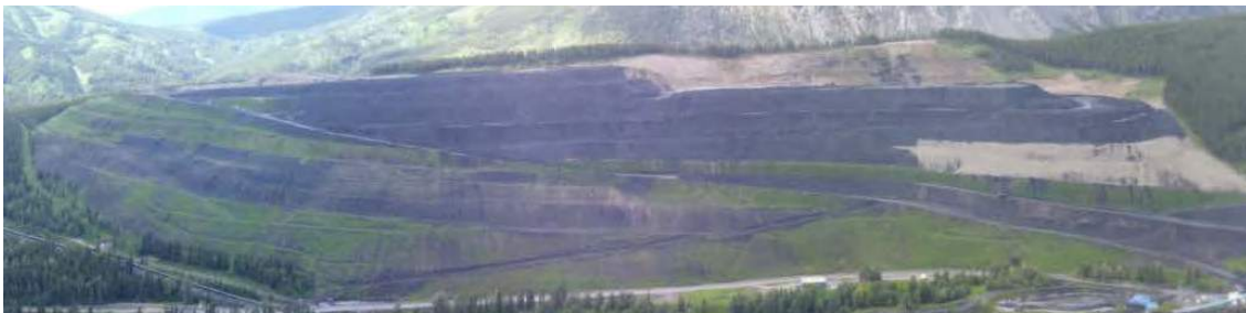
Figure 6. Example of progressive reclamation concurrent with operations for a mine waste dump.
