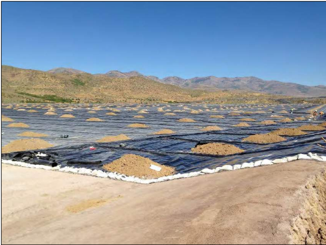
Figure 20. Ballast placement during liner installation
