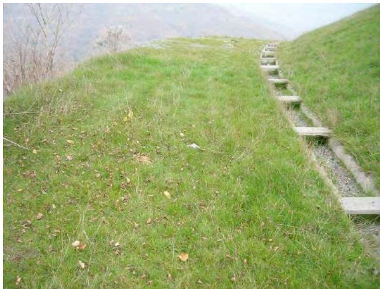
Fig. 6: Runoff collection channel on a top berm. Grass has already covered the remodeled sterile fills.
