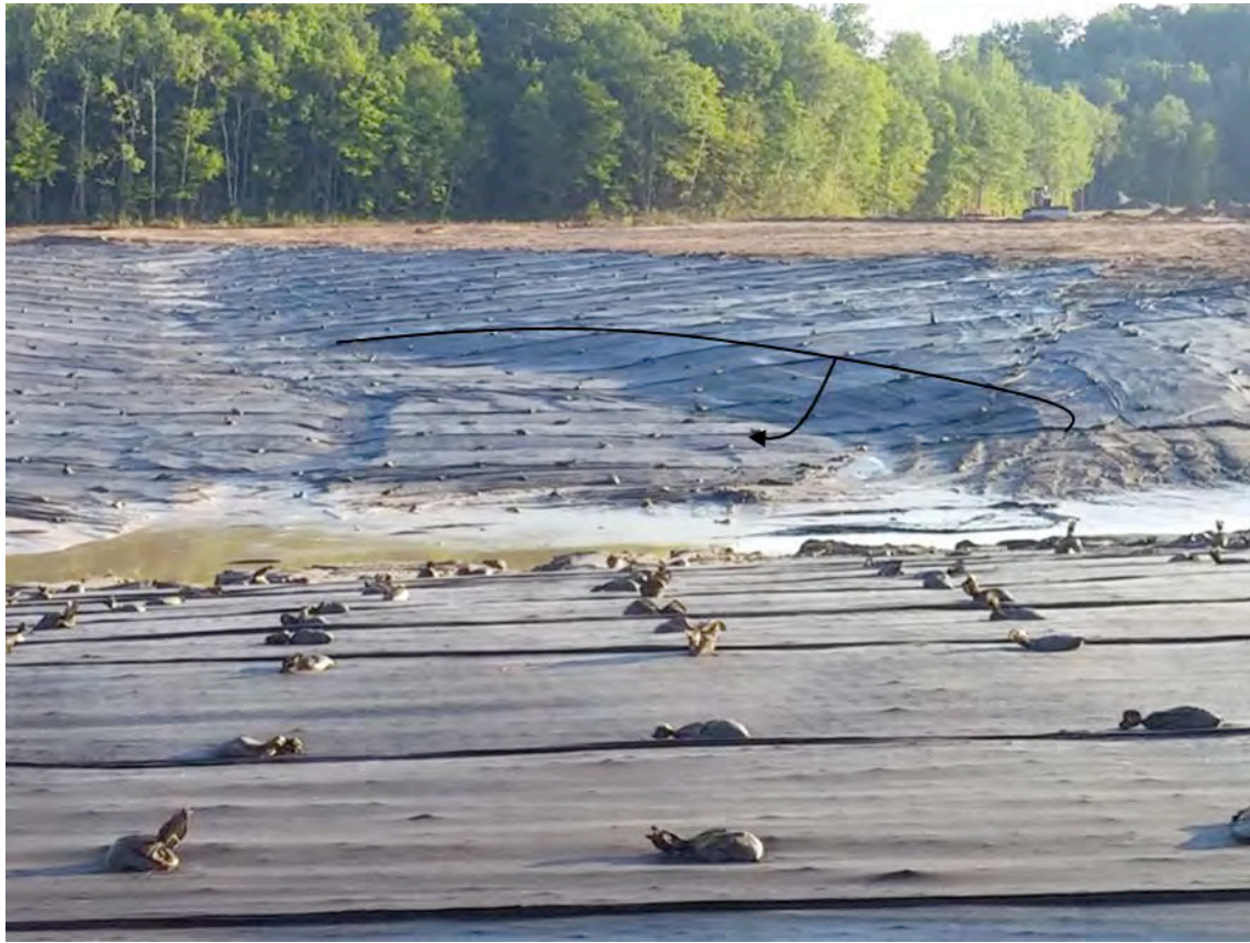
Figure 1. Photograph of the observed tailings sloughing in the lower swale.
