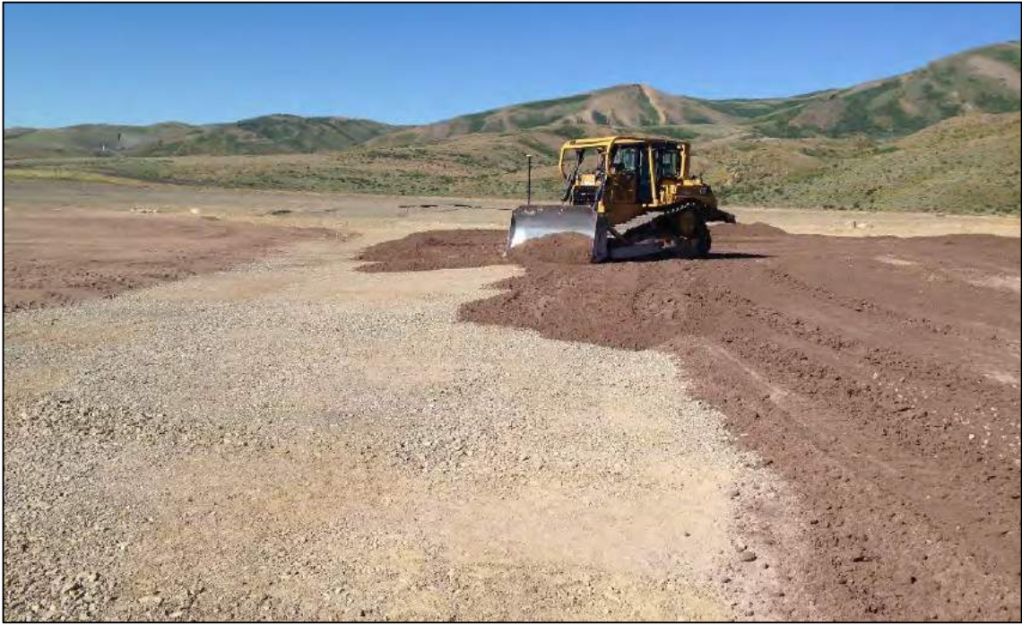
Figure 12. Capping IWP with dried tailings.
