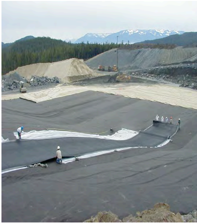
Figure 6 Typical Liner Placement
