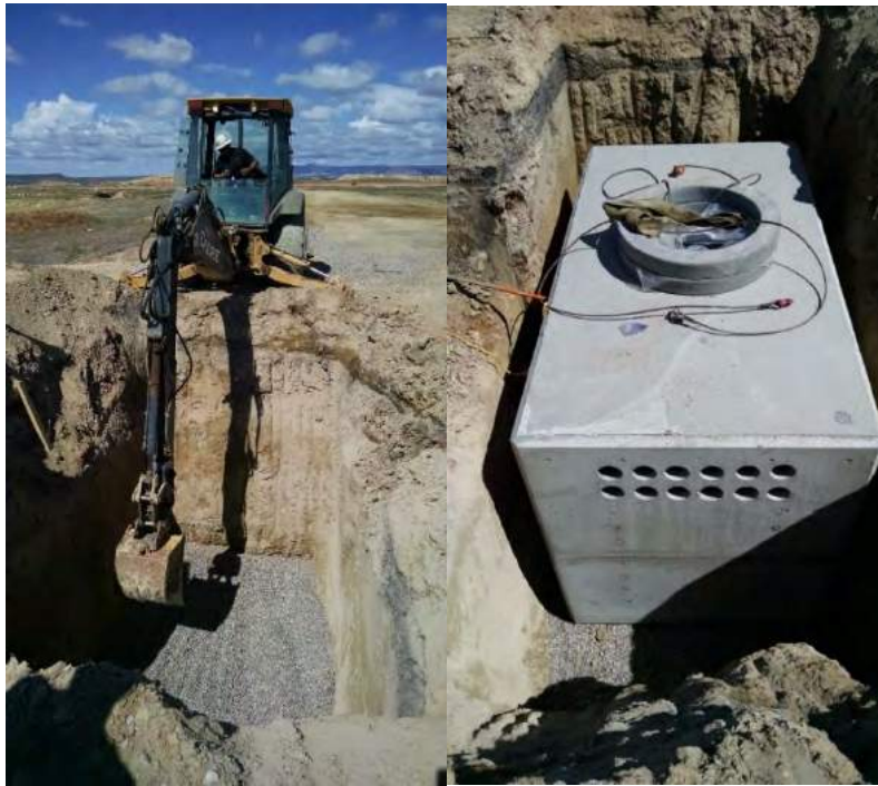
Figure 11. Excavation and placement of vault for monitoring basins.
