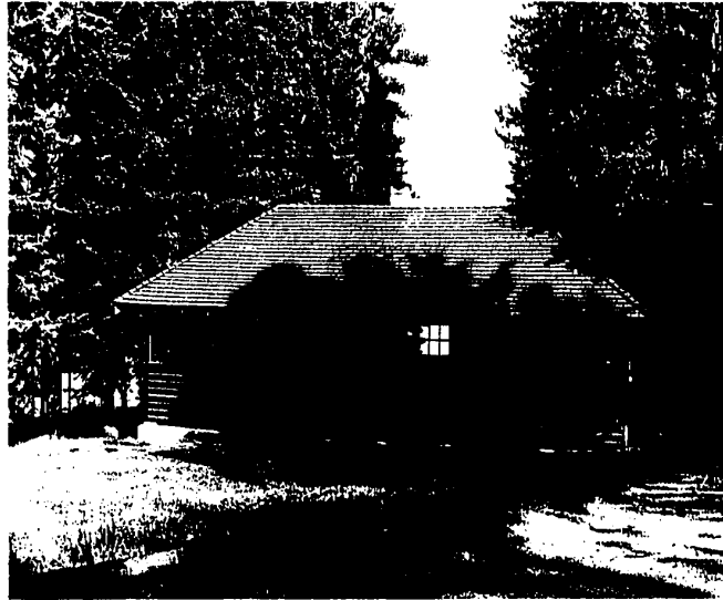
Figure 14. Kitchen shelter at Mt. Kerkeslin.
