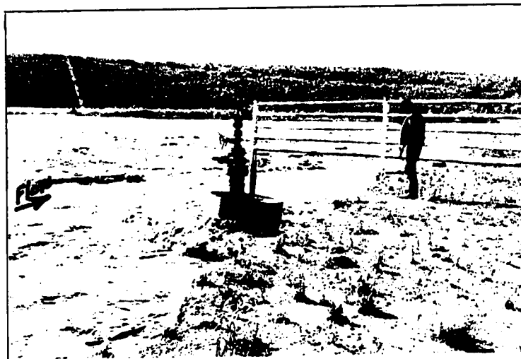
(b) Water injection well being eroded Revetment completely failed. June 19, 1965 - 4:30pm. Q \approx 47,000 cfs.
