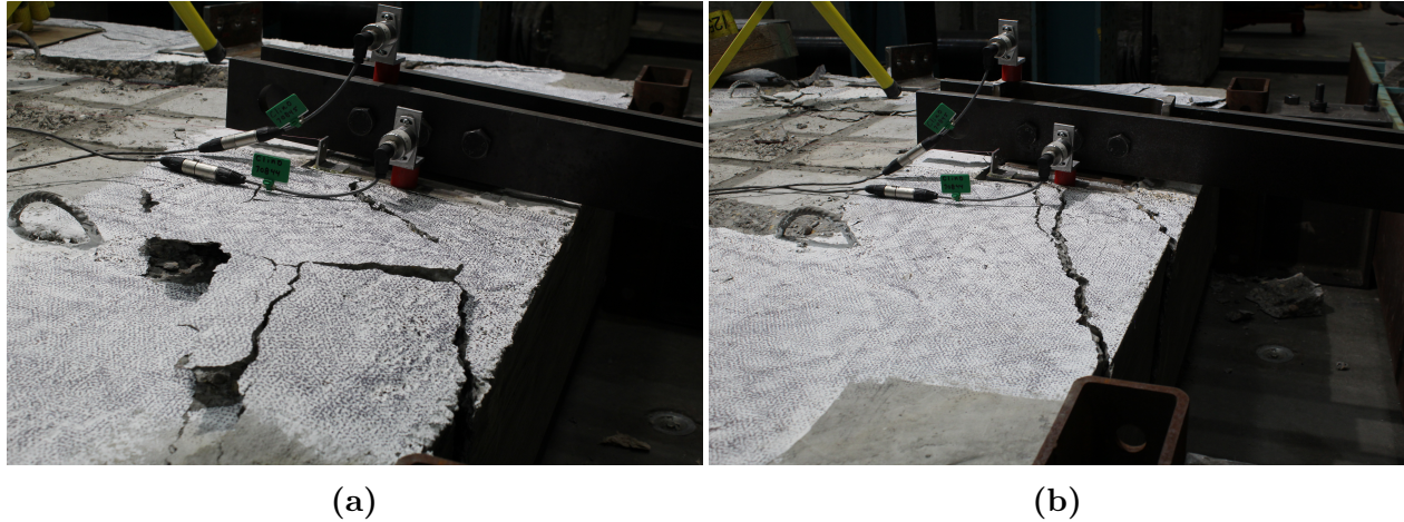
Figure 6.16 – Failure surfaces of (a) ST-215 B and (b) DA-215 B
