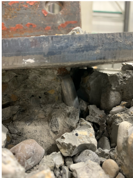
Figure 6.11 – Back stud of DA-215 B which yielded due to bending, but also experienced notable shear deformation just below the weld that connected it to the baseplate.
