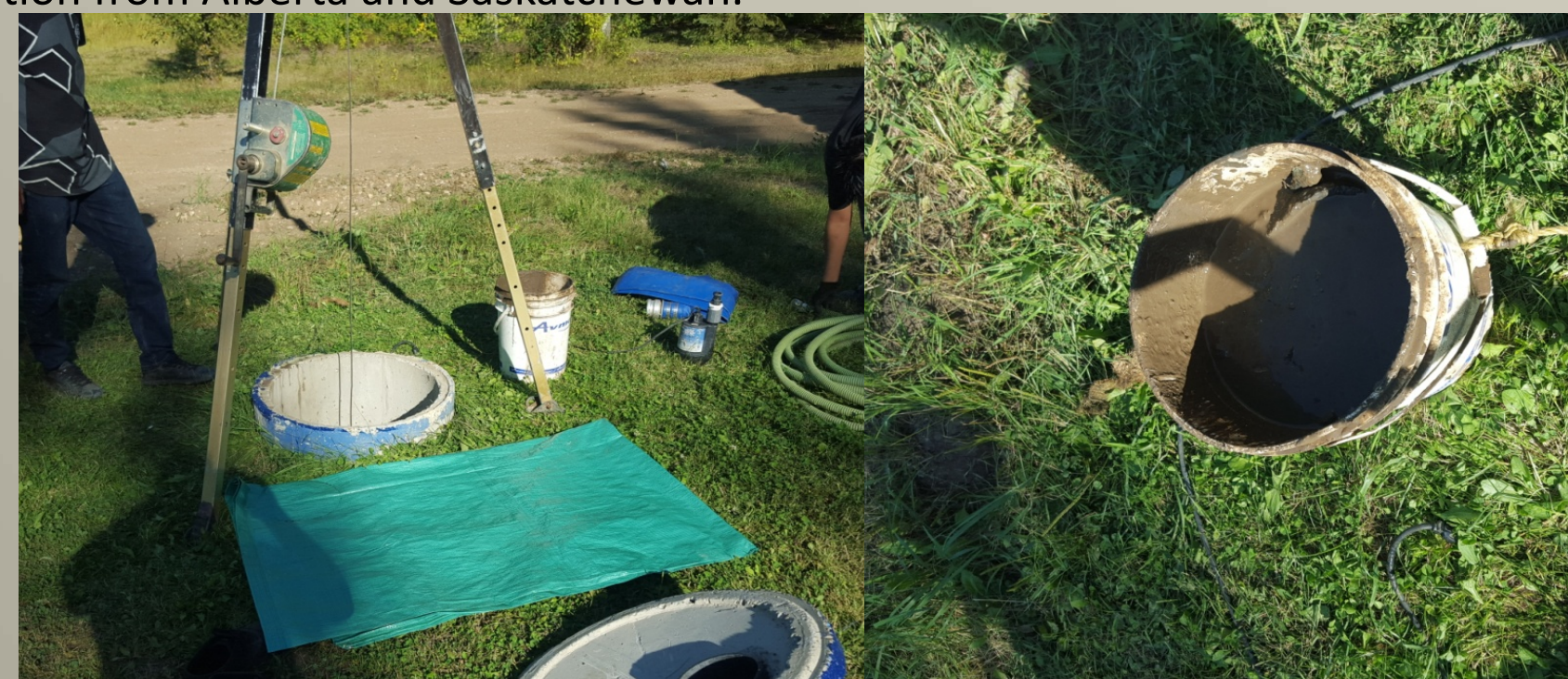
Cleaning of In ground drinking water cisterns in Chateh
