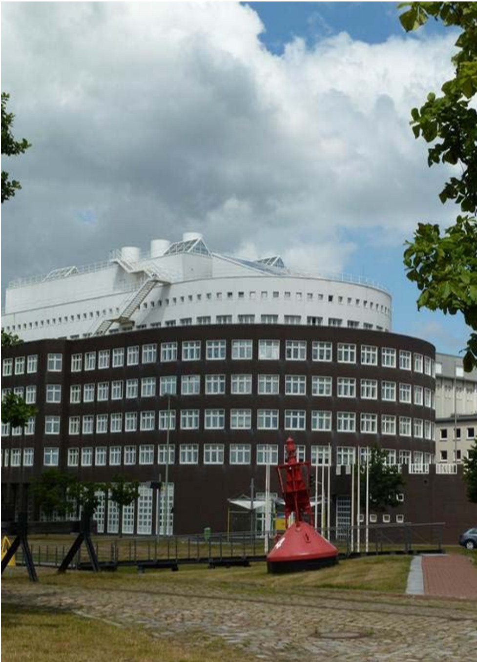
Figure 1: The AdP at the 5th floor of the Wegener-building at Bremerhaven, photo by C. R. Salewski
