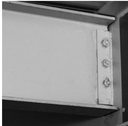
Figure 1-1: Typical shear tab Source: www.microstran.com.au
