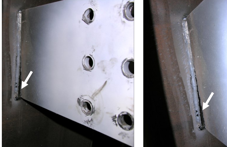
Figure 3-13: Weld rupture in specimen 3BM-13-0
