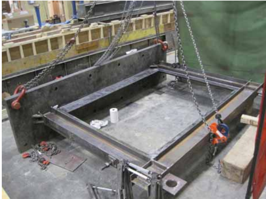
Figure 6-12: Rigid Frame Laid Down Flat for Infill Panel Installation
