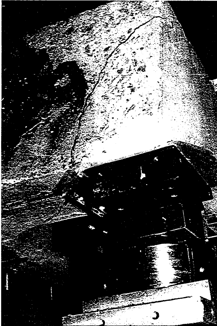
Figure A.8 Typical Round End Diaphragm Crack
