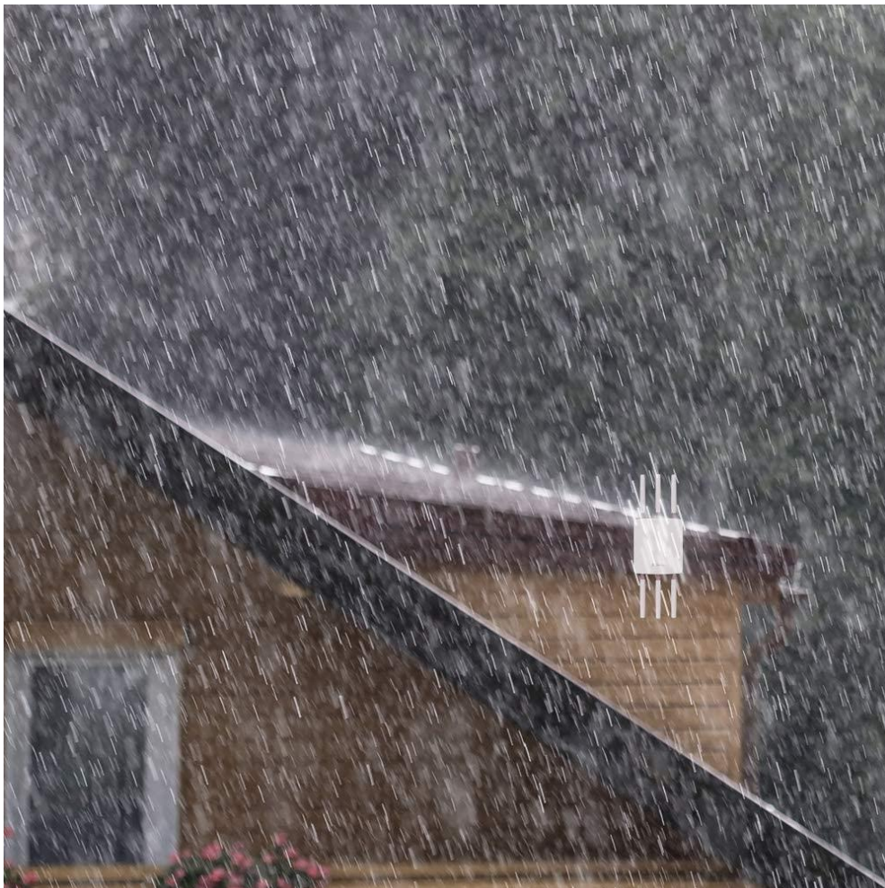
Figure 24 Wireless Access Point placed outside in the rain [25]
