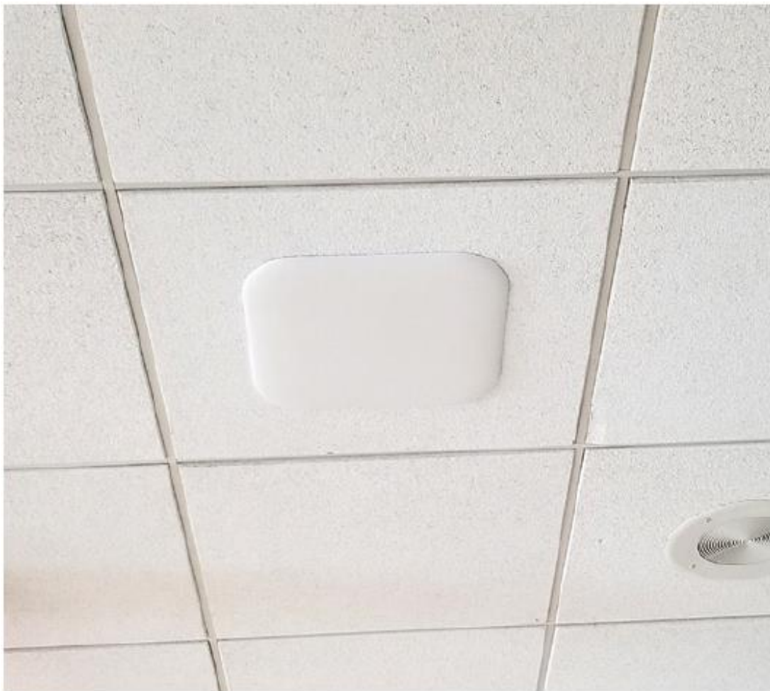
Figure 27 The goal accomplished is to install the AP in a low-profile ceiling mount while still using the original tile. [30]
