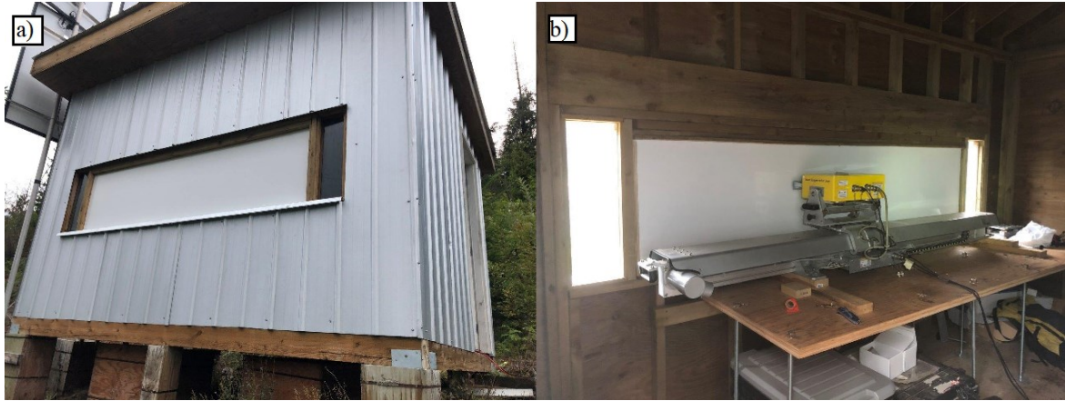
Figure 3-6: Protective Rohacell foam window as viewed from outside shelter a) and inside shelter b)
