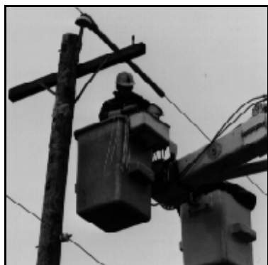
Installing Hawk Roosting Bars
