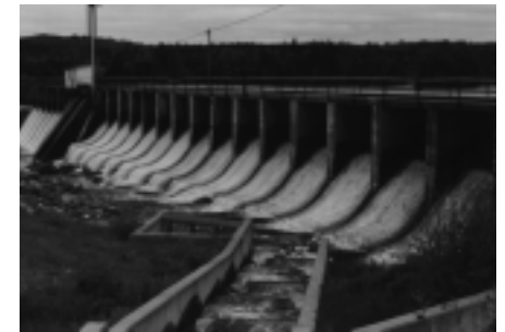
Fish Ladder at Ruth Falls, Sheet Harbour
